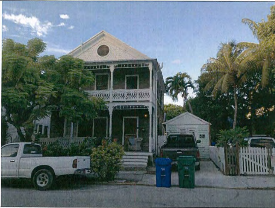
10. 408 Elizabeth Street. View from Elizabeth Street.
