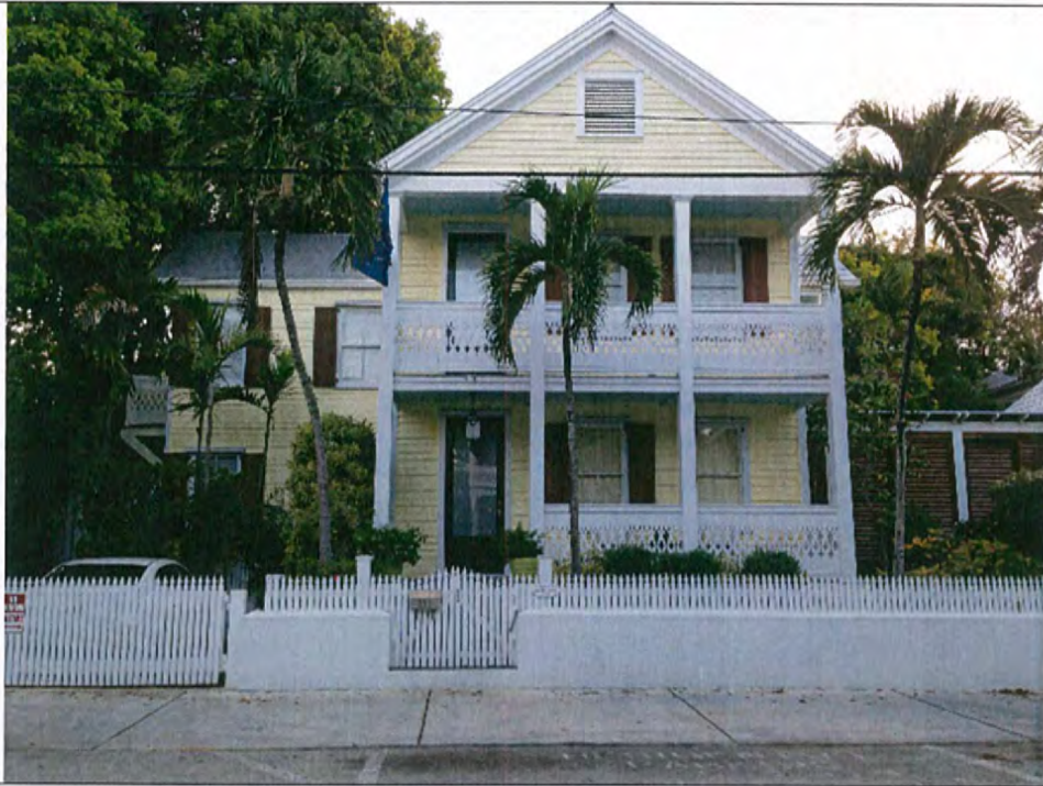
9. 411 Elizabeth Street. View from Elizabeth Street.
