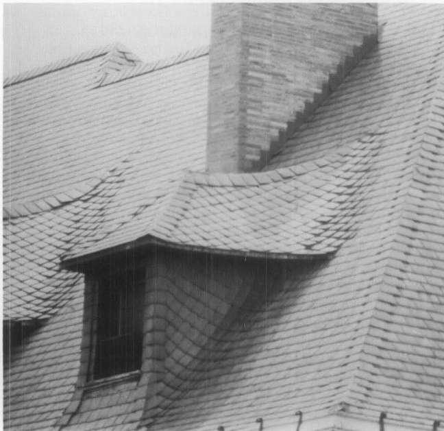
Because of the roof's visibility, the slate detailing around the dormers is important to the character of this structure. Note how the slates swirl from a horizontal pattern on the main roof to a diamond pattern on the dormer roofs and side walls. (18th and Que Streets, NW, Washington, D.C.)
