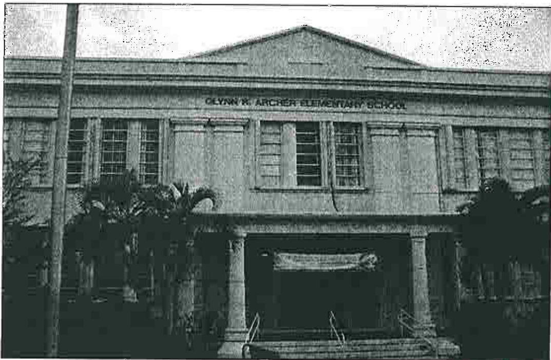
Photograph 2 shows the front of the main building
