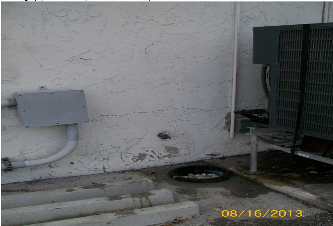
Drainage pipe on left in photo drains to asphalt below.
