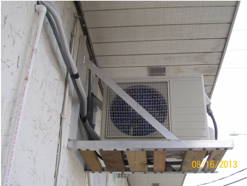
Drainage pipe on left in photo drains to asphalt below.
