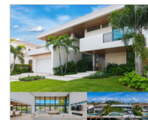
Solar Isles Residence
