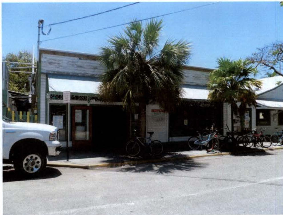
404 SOUTHARD STREET - EXISTING WEST BUILDING
