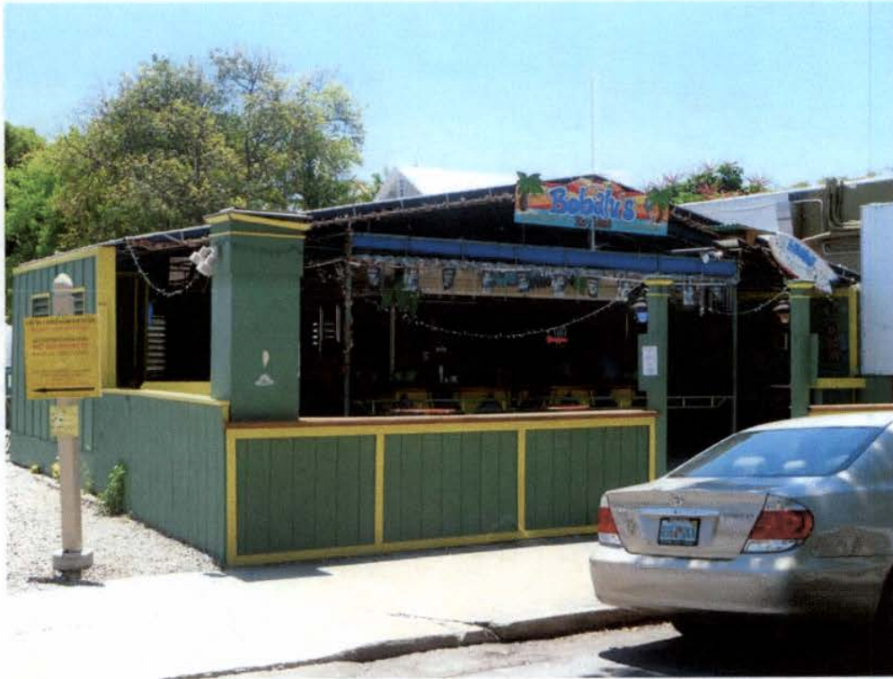
404 SOUTHARD STREET - EXISTING EAST BUILDING
