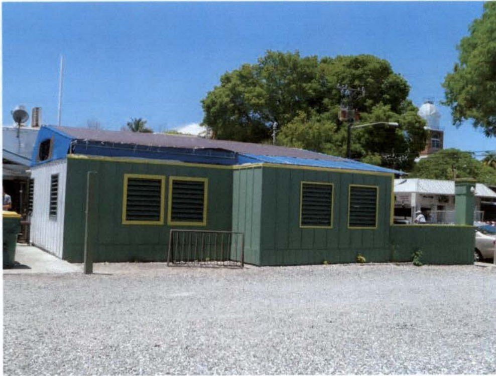
404 SOUTHARD STREET - EAST BUILDING (EAST ELEVATION)
