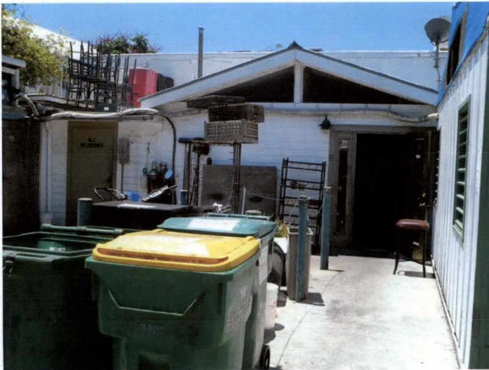
404 SOUTHARD STREET - REAR OF EAST BUILDING
