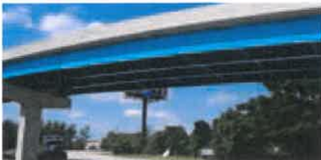
A typical roadway overpass prior to scanning with the ScanStation.
