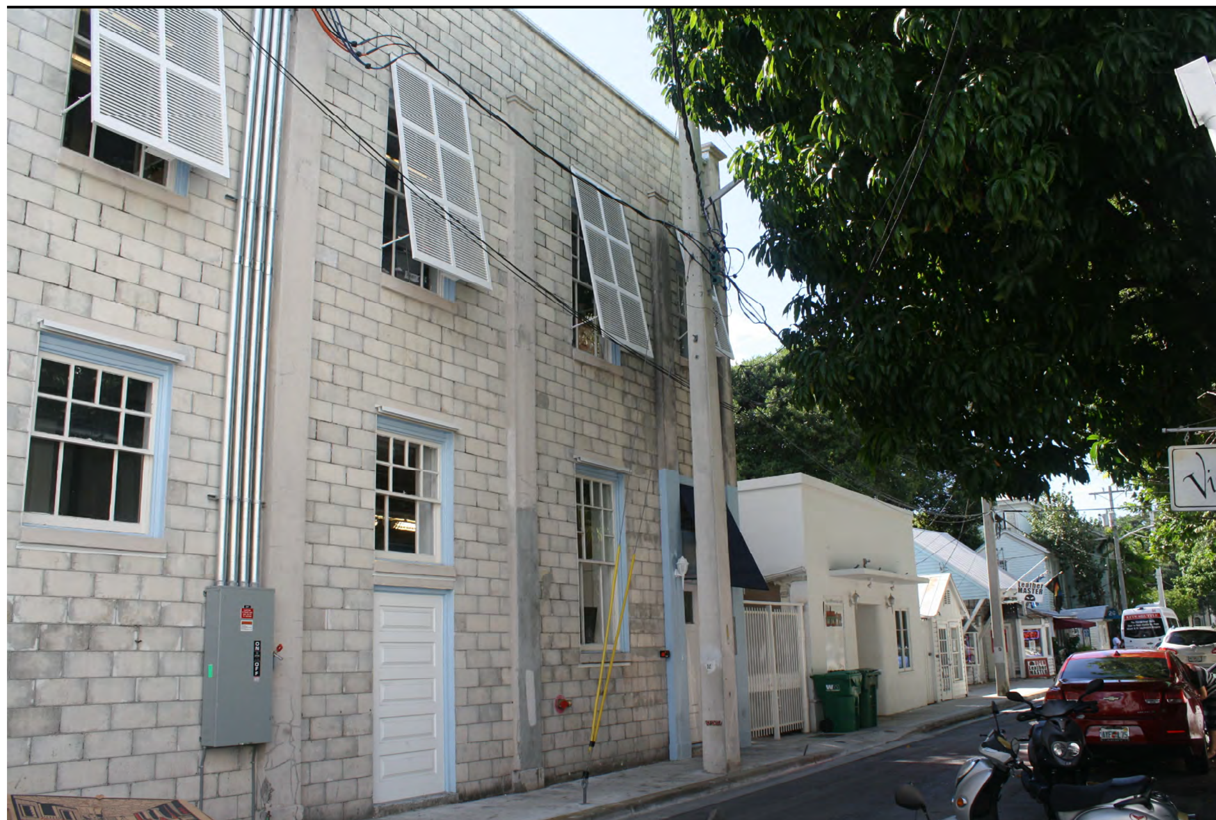
3 EX2 VIEW OF ADJACENT PROPERTY (TO NORTH OF 420-422 APPELROUTH LANE)
