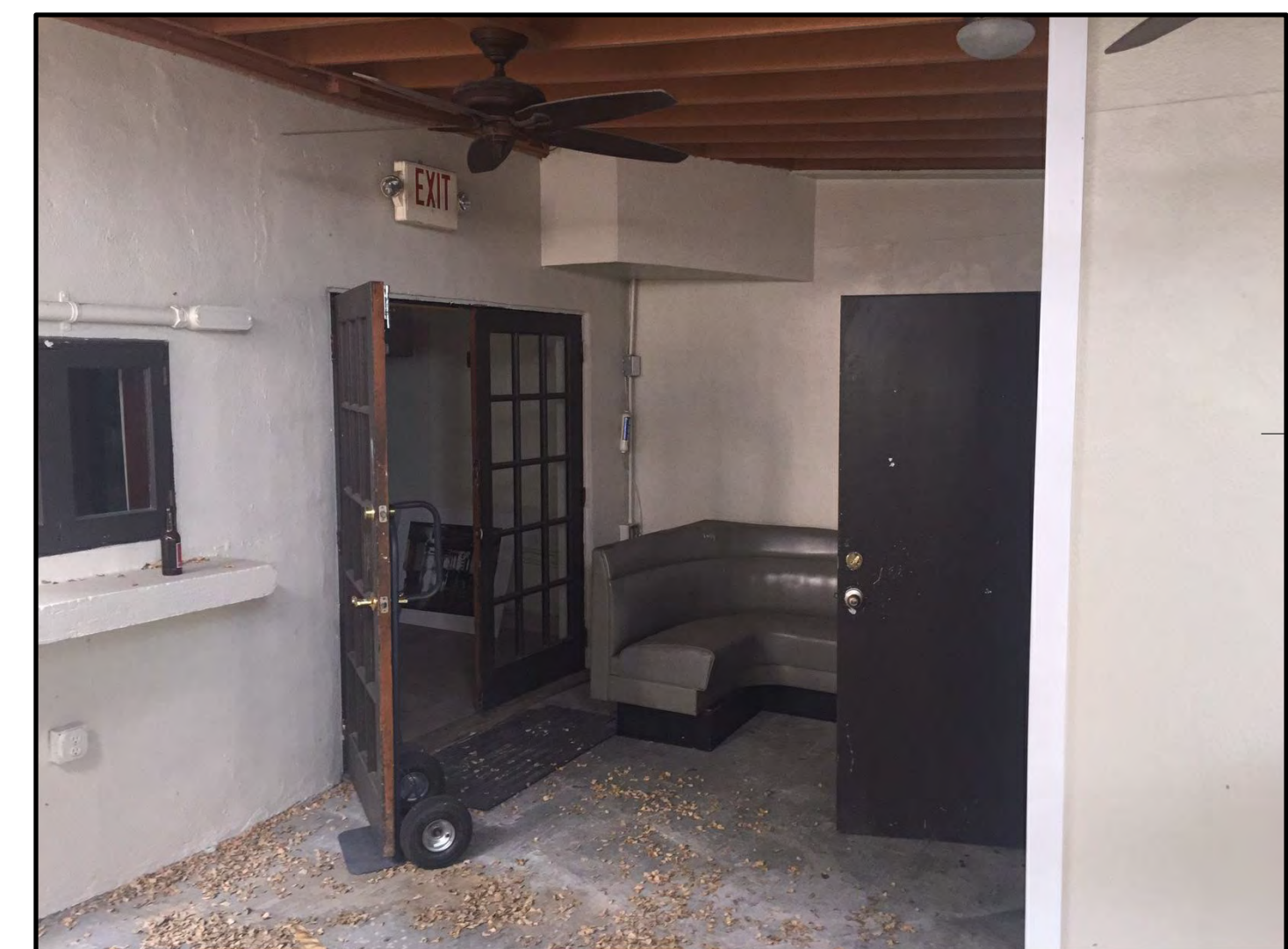
4 EX2 SEE DEMOLITION PLAN FOR PHOTO LOCATION
