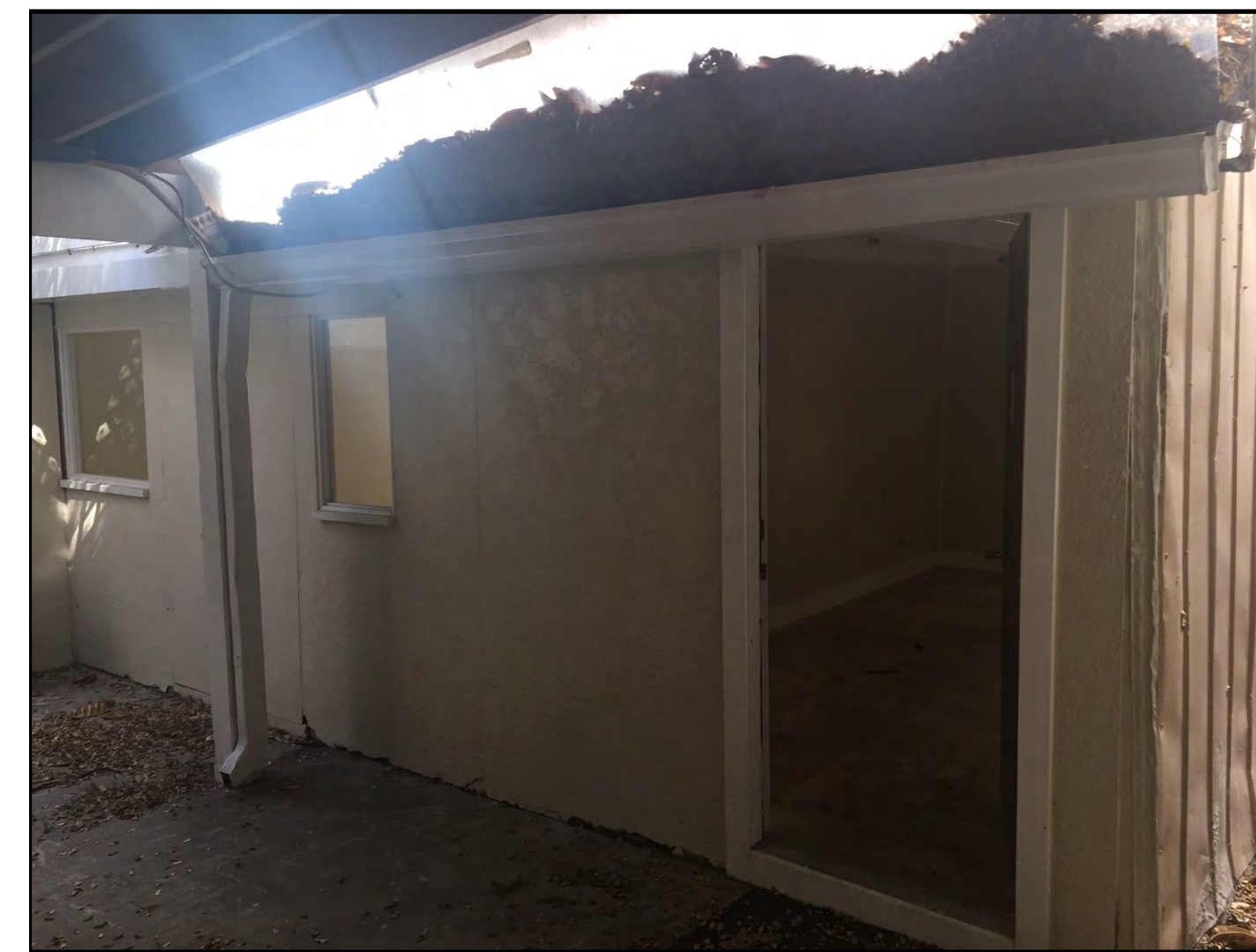
5 EX2 SEE DEMOLITION PLAN FOR PHOTO LOCATION
