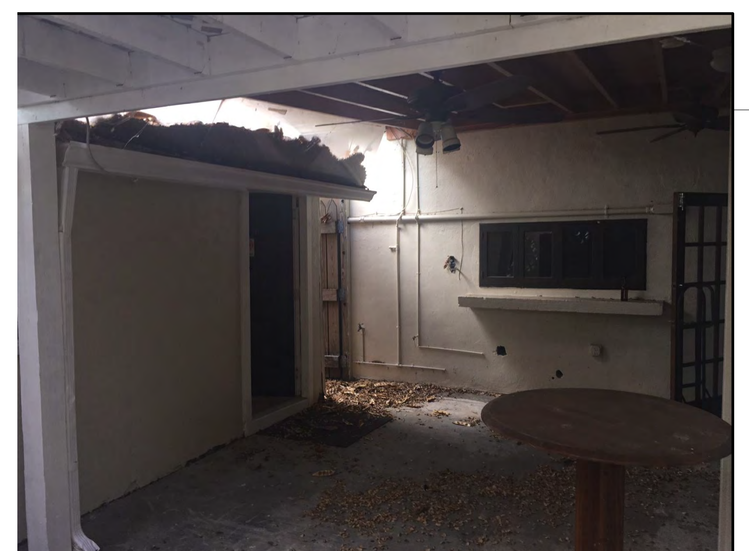
1 EX2 SEE DEMOLITION PLAN FOR PHOTO LOCATION
