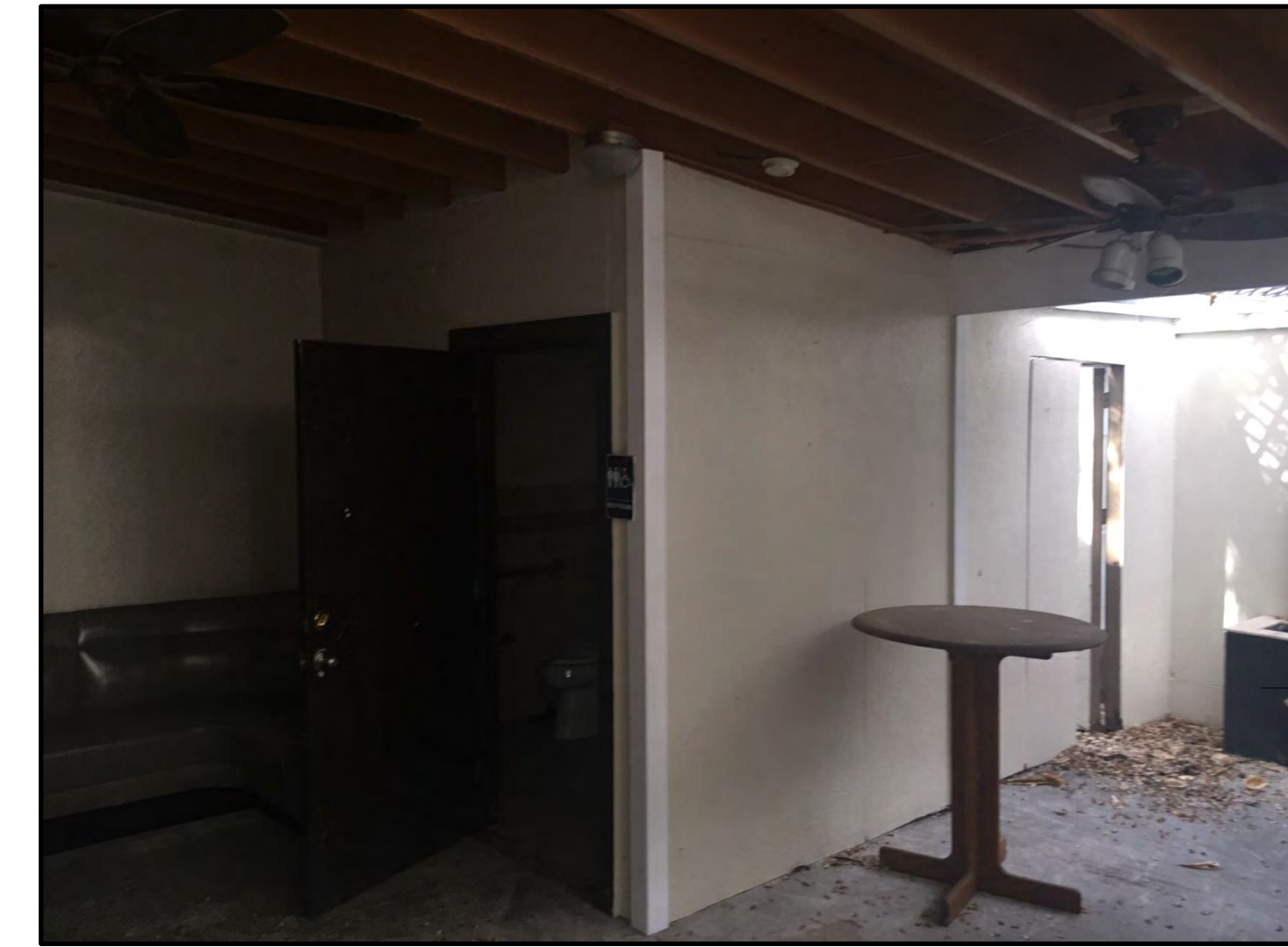
7 EX2 SEE DEMOLITION PLAN FOR PHOTO LOCATION
