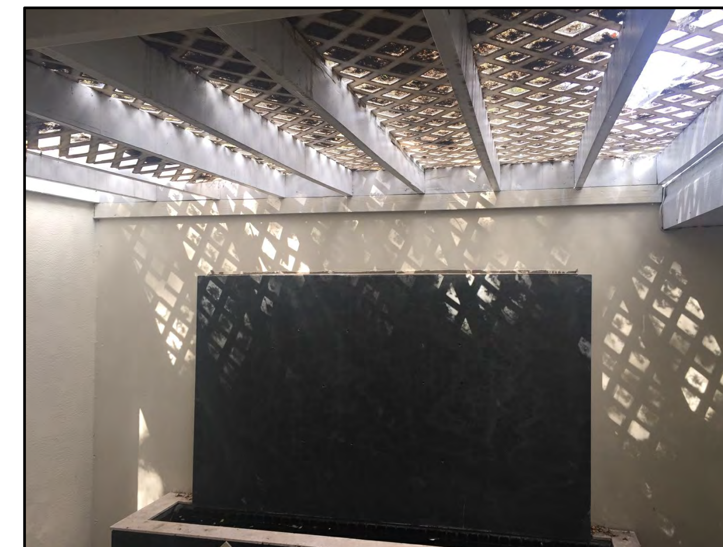
2 EX2 SEE DEMOLITION PLAN FOR PHOTO LOCATION
