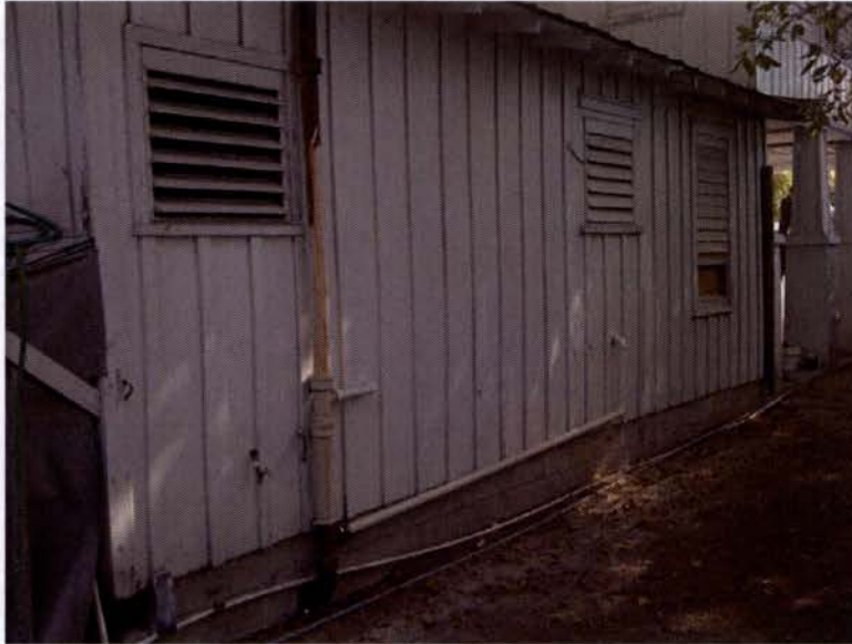
SOUTH WEST SIDE OF HOUSE LOOKING TOWARDS THE FRONT
