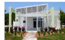
Lantana Police Annex
