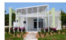
Lantana Police Annex
