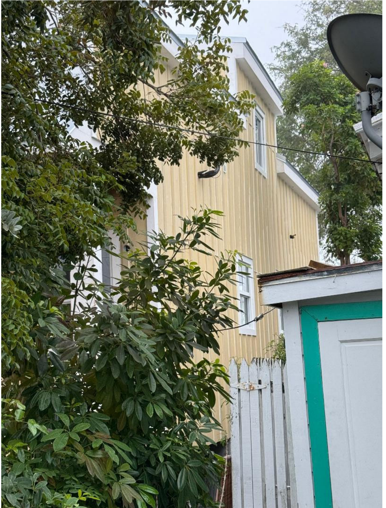
318 Amelia - New Construction , two AC units
