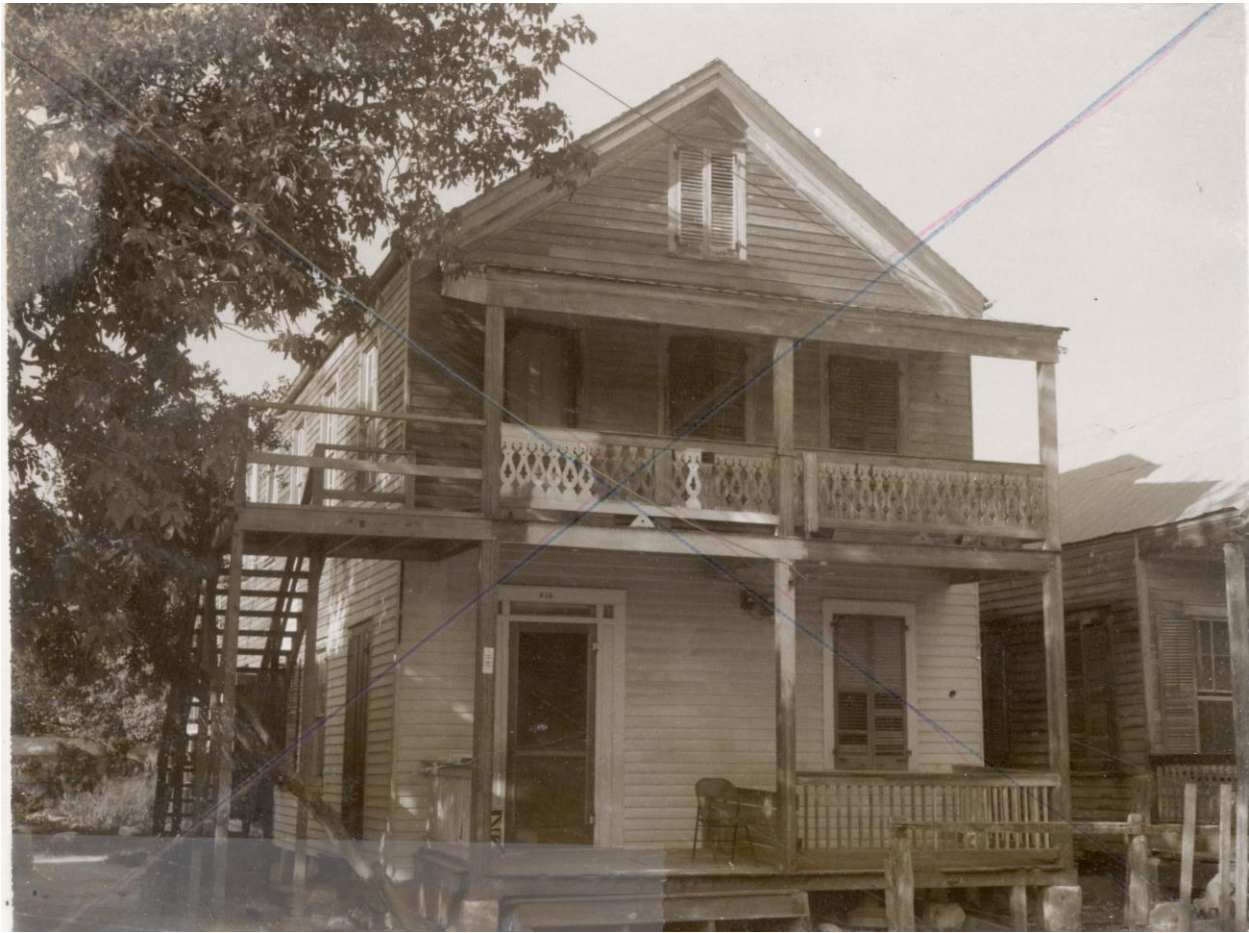
1965 photo of the two-story structure that once fronted 914 Thomas Street. The structure was razed in 1973.
