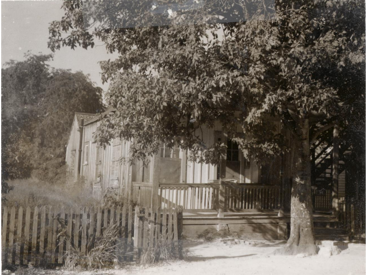
1965 photo of the one-story structure at 916 Thomas Street. The structure that stood directly behind it at 916½ Thomas Street was razed sometime between 1948 and 1962.
