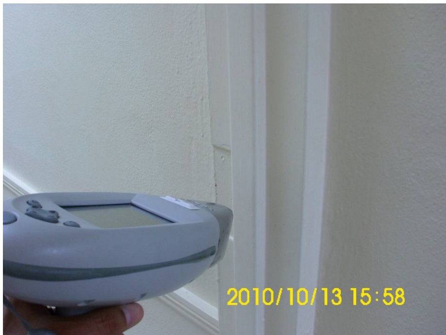
Photograph #4: Interior LBP metal door jamb/casing tested with XRF and sampled for lab analysis during this inspection.
