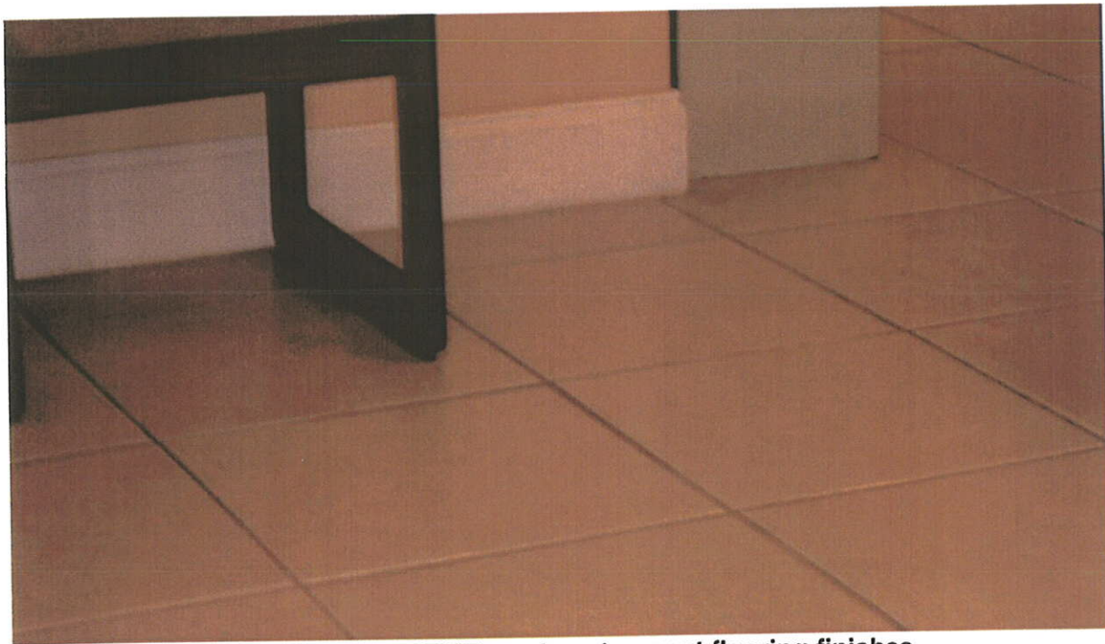
Photo 18: Floor 2 IT Department current flooring finishes
