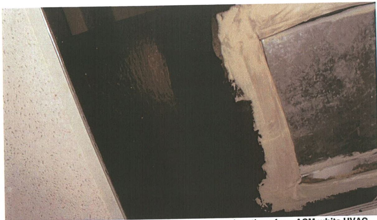
Photo 9: More ACM HVAC mastic above ceilings, at junction of nonACM white HVAC
