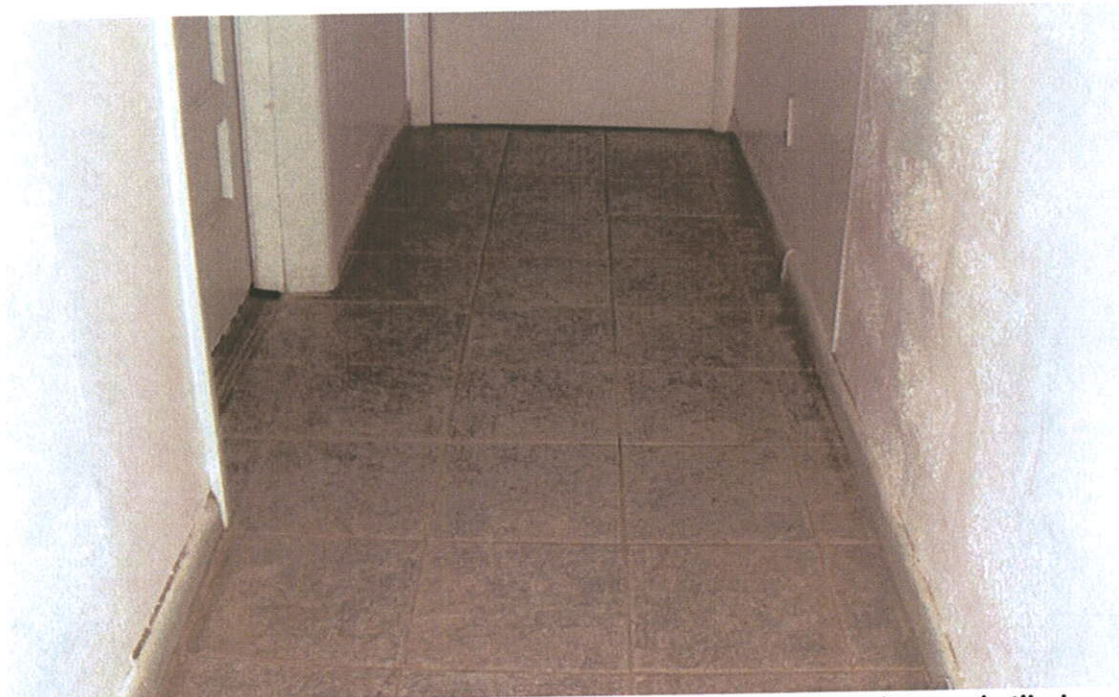
Photo 11: ACM VFT/mastic presumed present beneath floor 1 ceramic tiled areas
