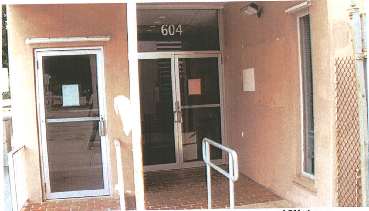
Photo 1: Entrance to Annex Building at 604 Simonton, nonACM stucco
