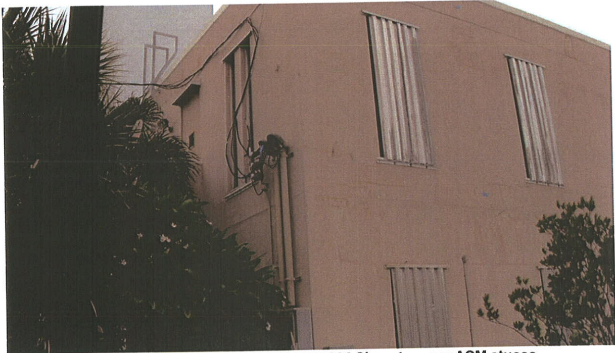
Photo 4: Side of Annex Building at 604 Simonton, nonACM stucco
