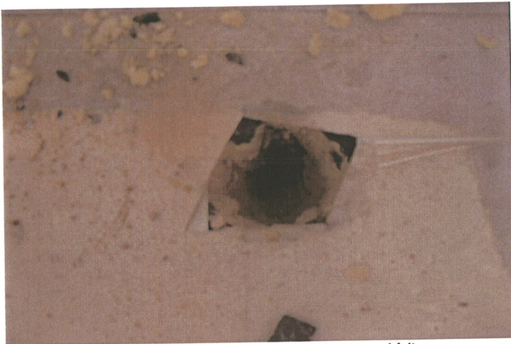
Photo 14: NonACM roof field membrane and felts
