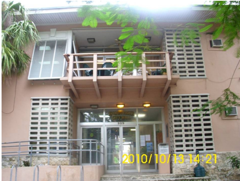
Photograph #1: Key West City Hall building – 525 Angela Street, Key West, FL
