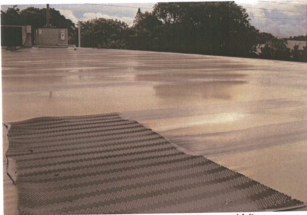
Photo 13: NonACM roof field membrane and felts
