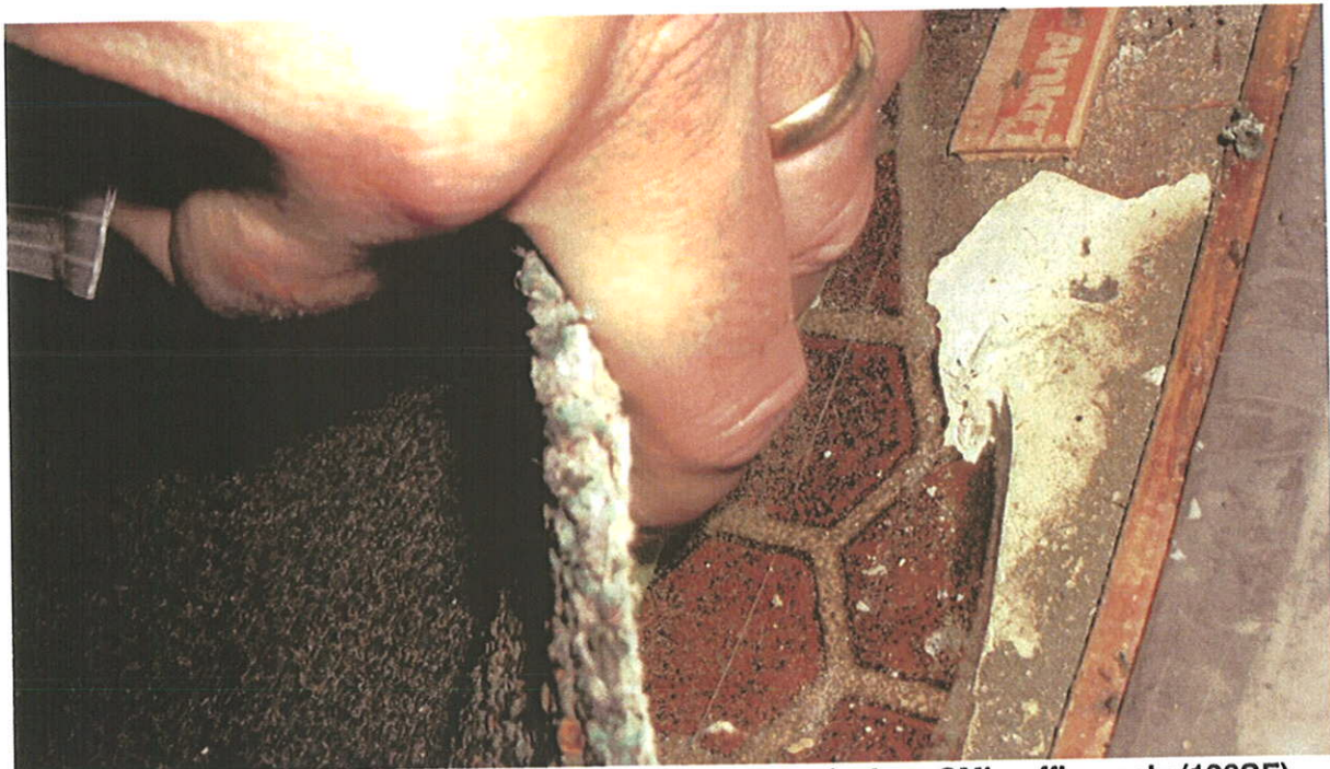
Photo 20: ACM redbrick lino identified under carpet in Ass. CM's office only (120SF)
