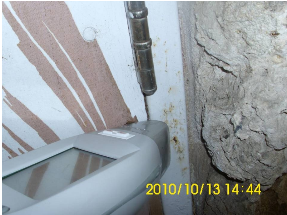
Photograph #3: Exterior LBP metal door jamb/casing tested with XRF and sampled for lab analysis during this inspection.
