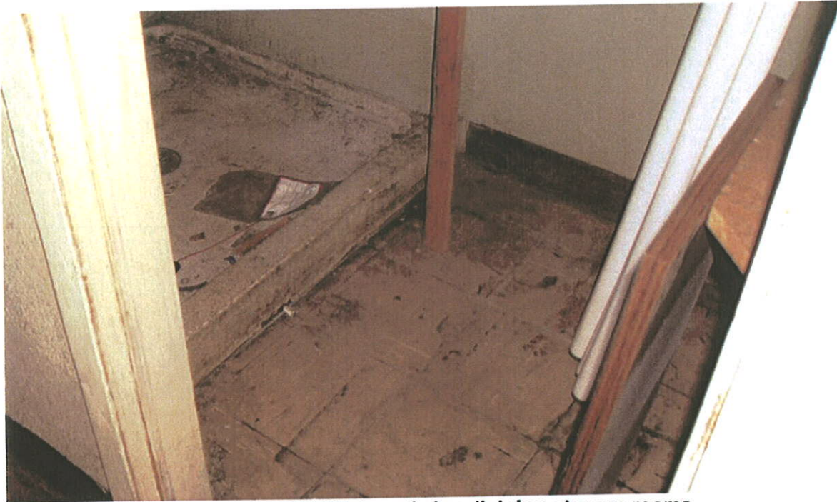
Photo 5: ACM VFT/mastic in adjoining storage rooms
