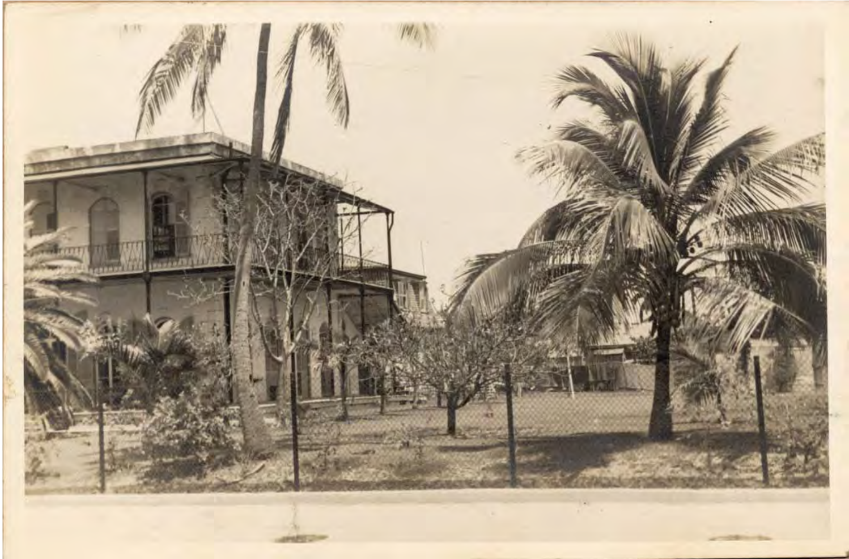
#907 Whitehead Street in the 1930's photo taken from Whitehead Street. Monroe County Library. The Heritage House Collection.
