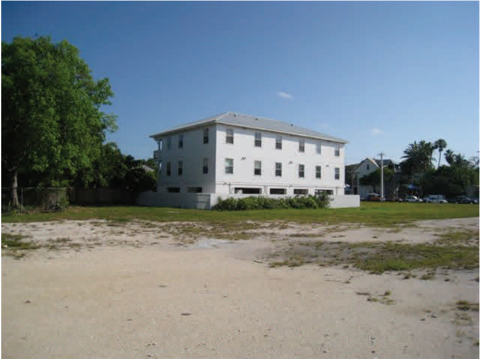
VIEW FROM SITE LOOKING SOUTH TO APARTMENT
