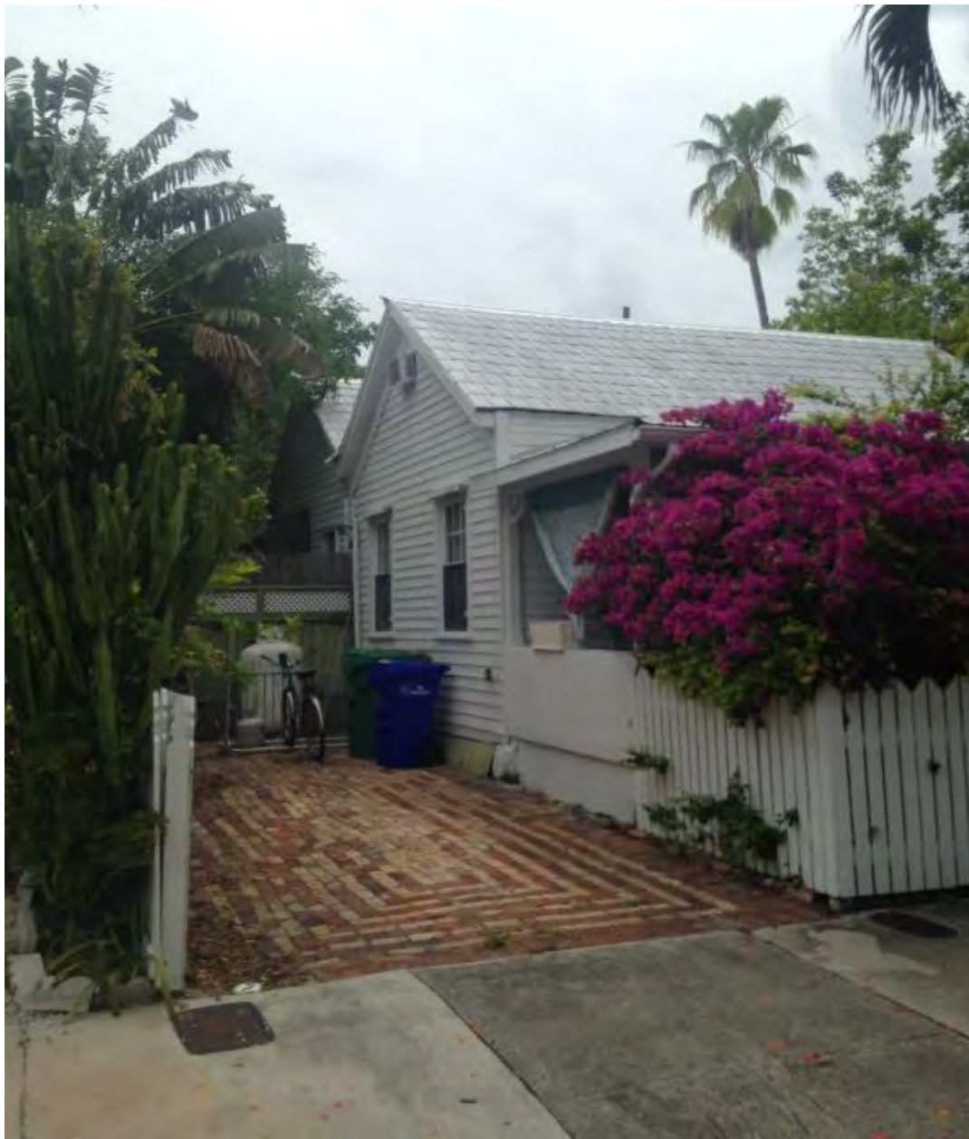
South side of house showing the two side gable roofs. These brick pavers will be removed.
