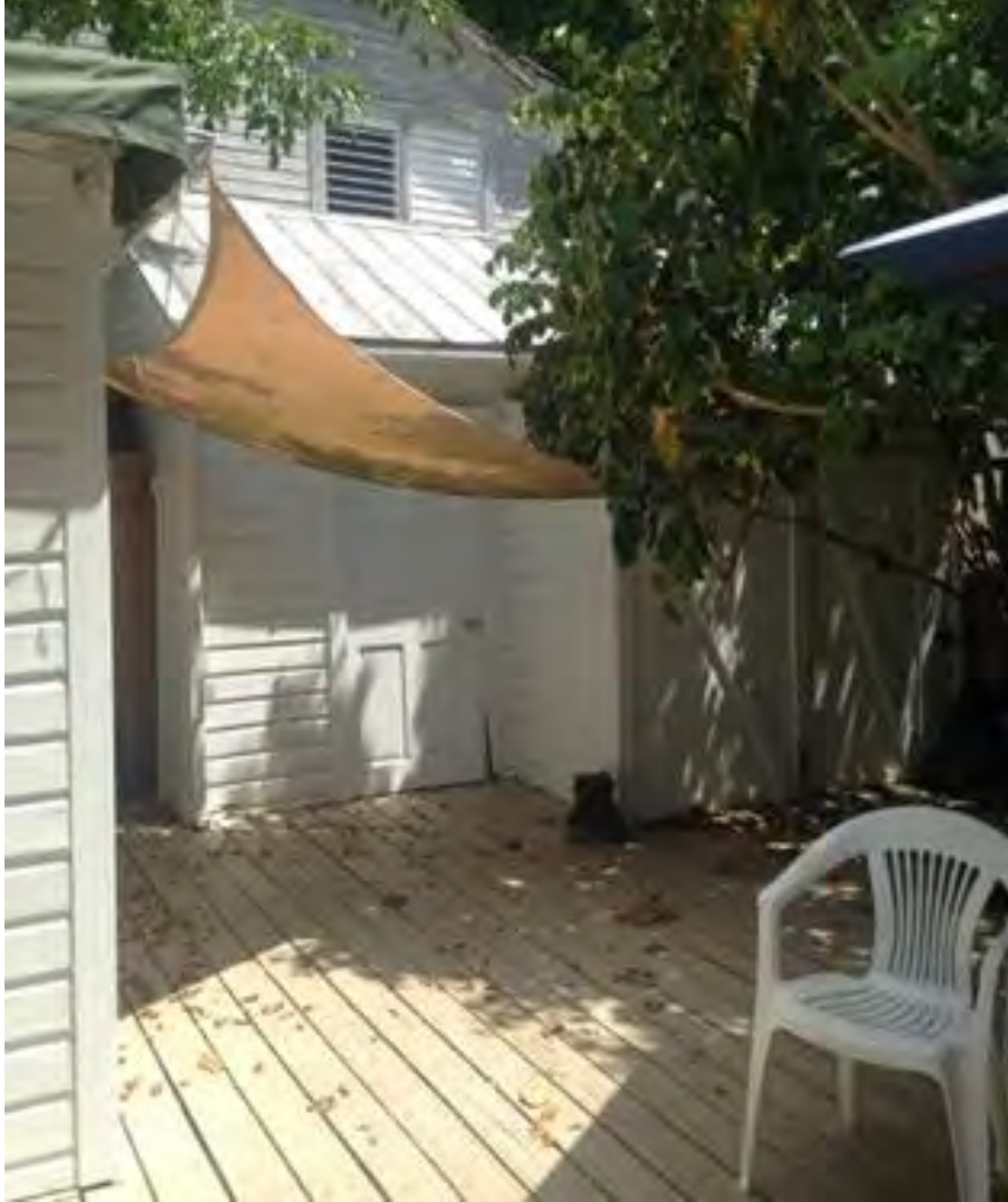
Shed on the right to be demolished.
