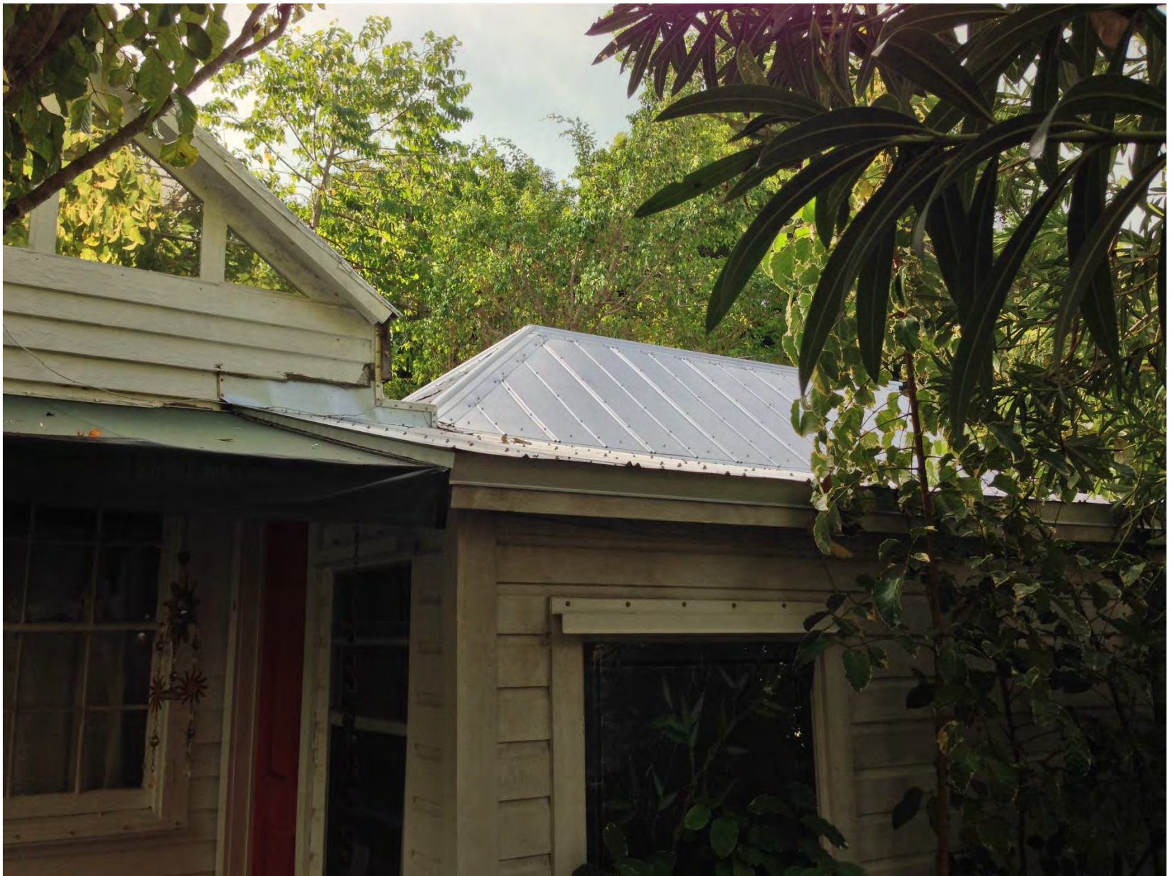
Roof that is hip in the front and gable in the rear. The V-Crimp roof is more recent.
