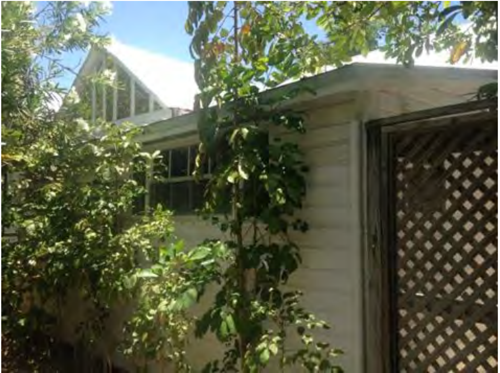
Another view of the south side of the house. Rear of the shed roof section that will be moved off city right-of-way.
