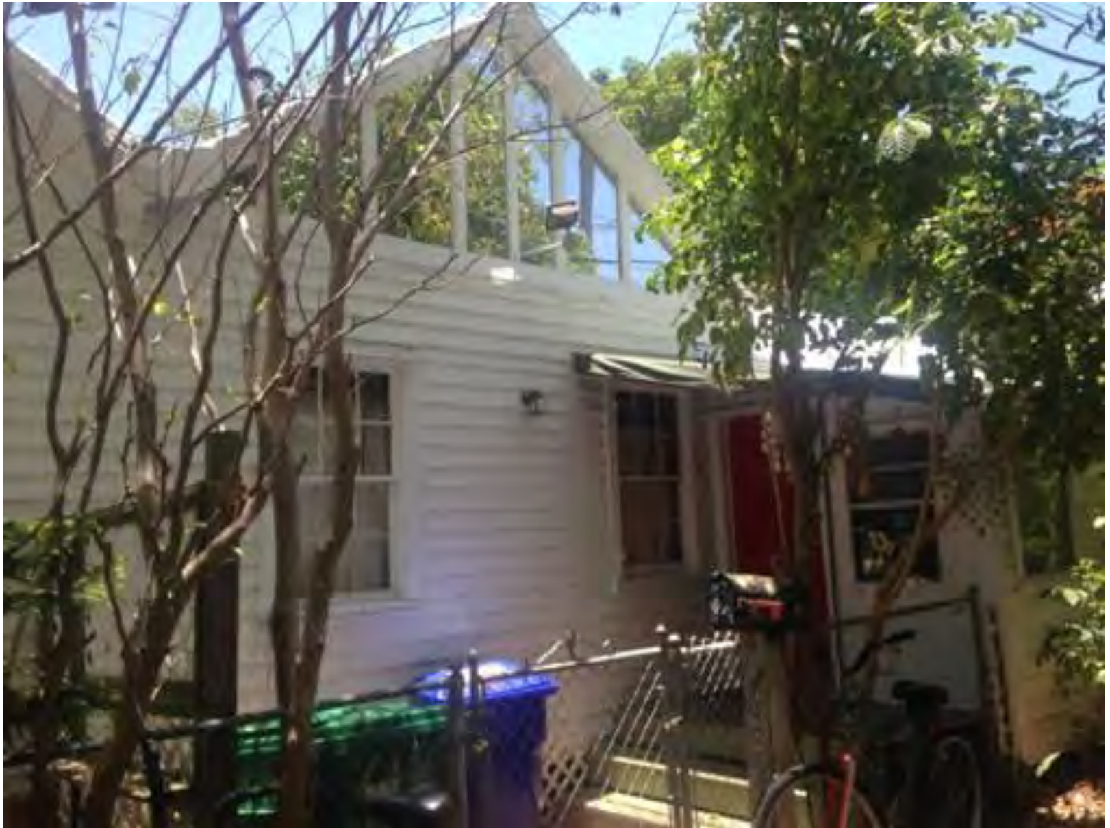
Inappropriate clerestory windows to be removed.
