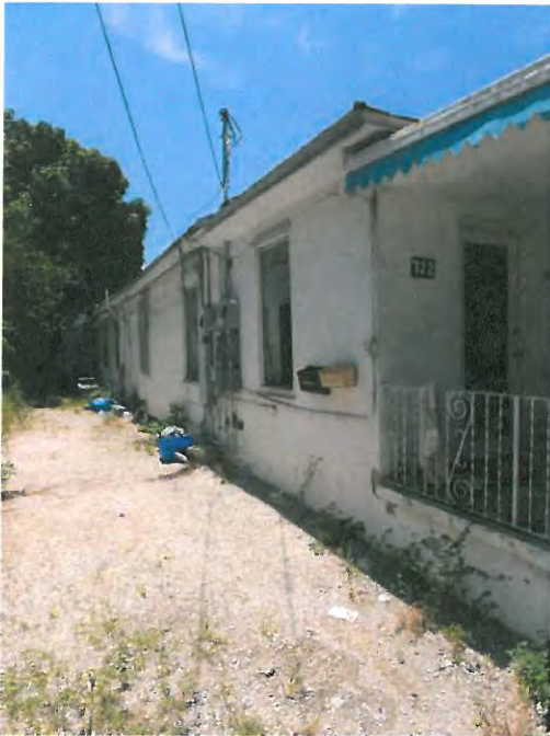
View of east side of main structure
