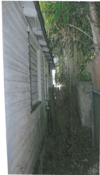
View of the east side of the secondary structure
