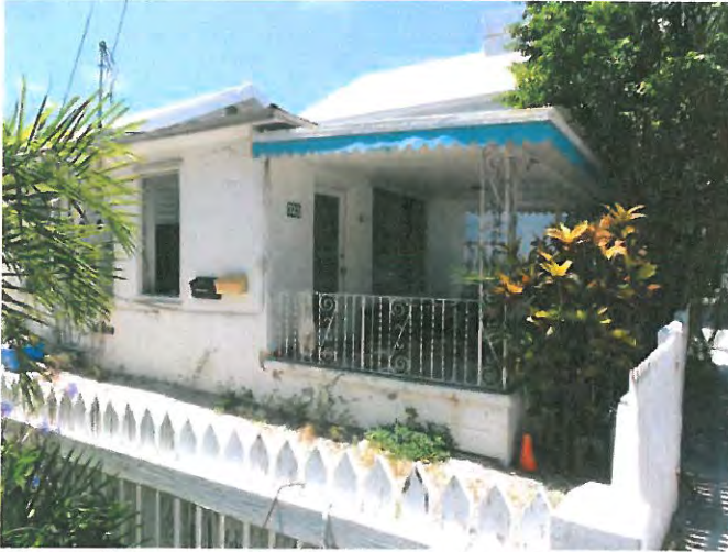
View of front porch of main structure along Caroline Street
