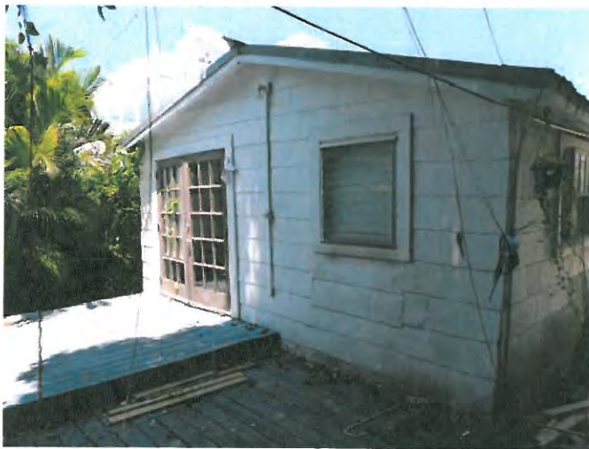
View of the rear of the main structure
