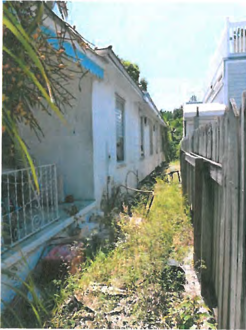
View of west side of main structure
