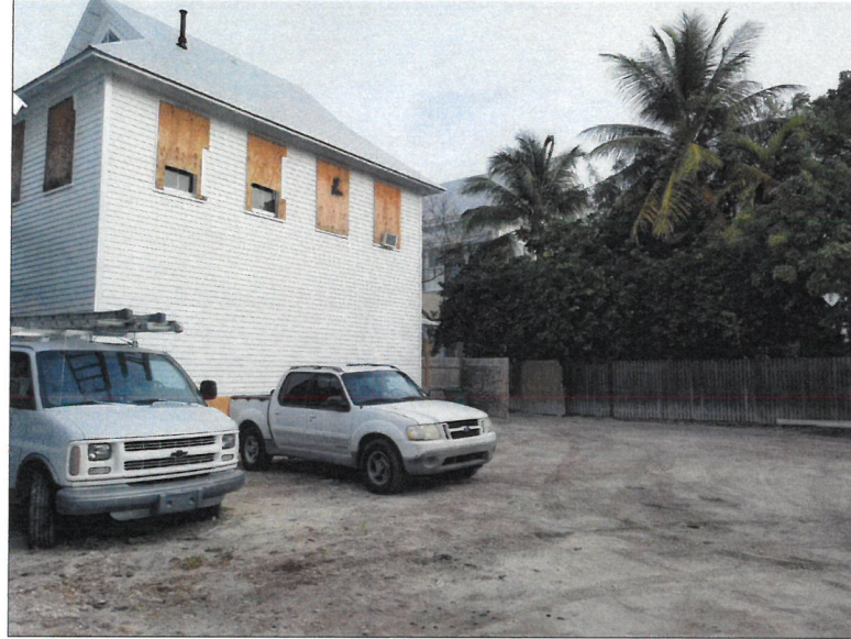
2 PHOTOGRAPH OF EXISTING SOUTH ELEVATION SCALE: N.T.S.
