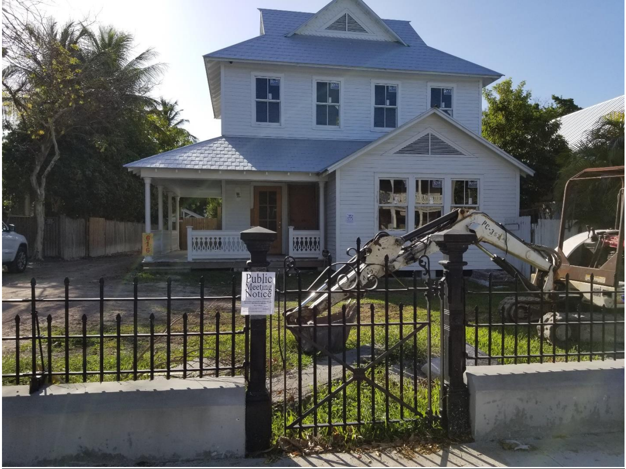
Photo of notice posted on fence at 616 Eaton Street.
