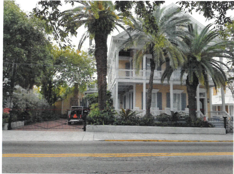
3 A9 PHOTOGRAPH OF ADJACENT PROPERTY TO THE EAST SCALE: N.T.S.
