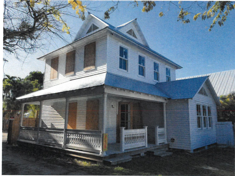
3 PHOTOGRAPH OF EXISTING EAST ELEVATION SCALE: N.T.S.
