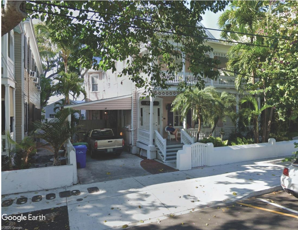
Photo from Google Earth showing the carport structure at 615 Fleming Street.
