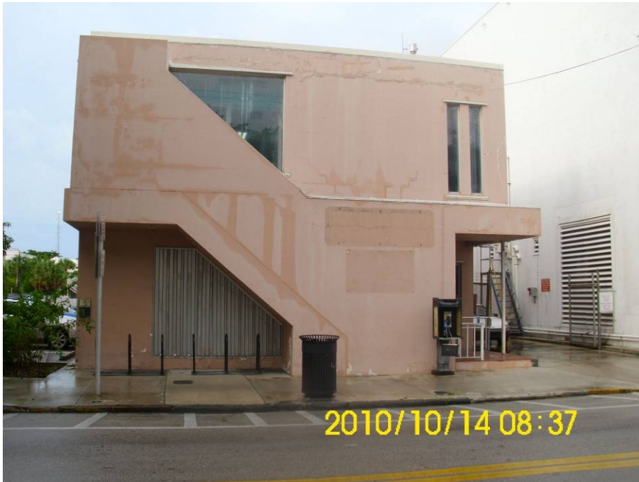
Photograph #5: Annex building – 604 Simonton Street, KW, Florida.
