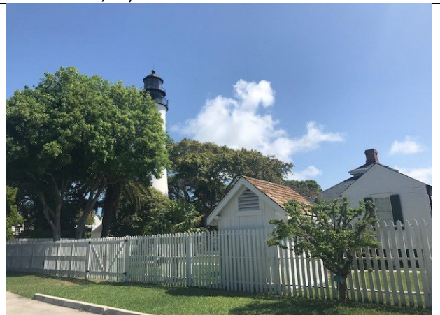
Historic Key West Lighthouse – Reproduce Fence & Gate/Repair Shed
