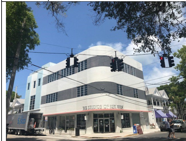
Studios of Key West – Water Intrusion Mitigation
