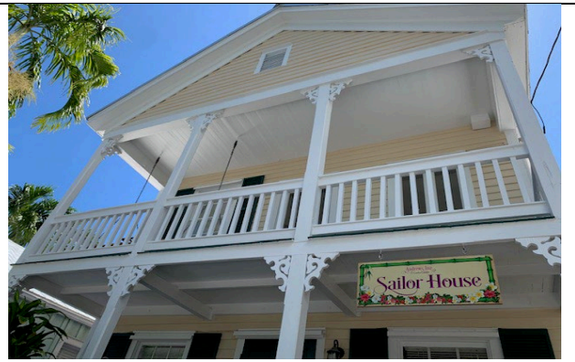
824 Center St., Key West – Interior Renovations
