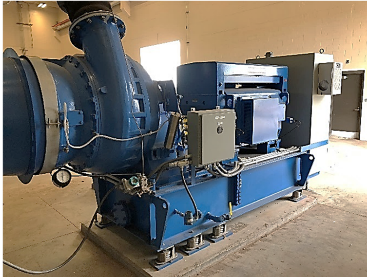
Figure 3-2: Single stage blower without enclosure
