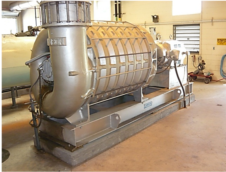
Figure 3-1: Multistage blower
