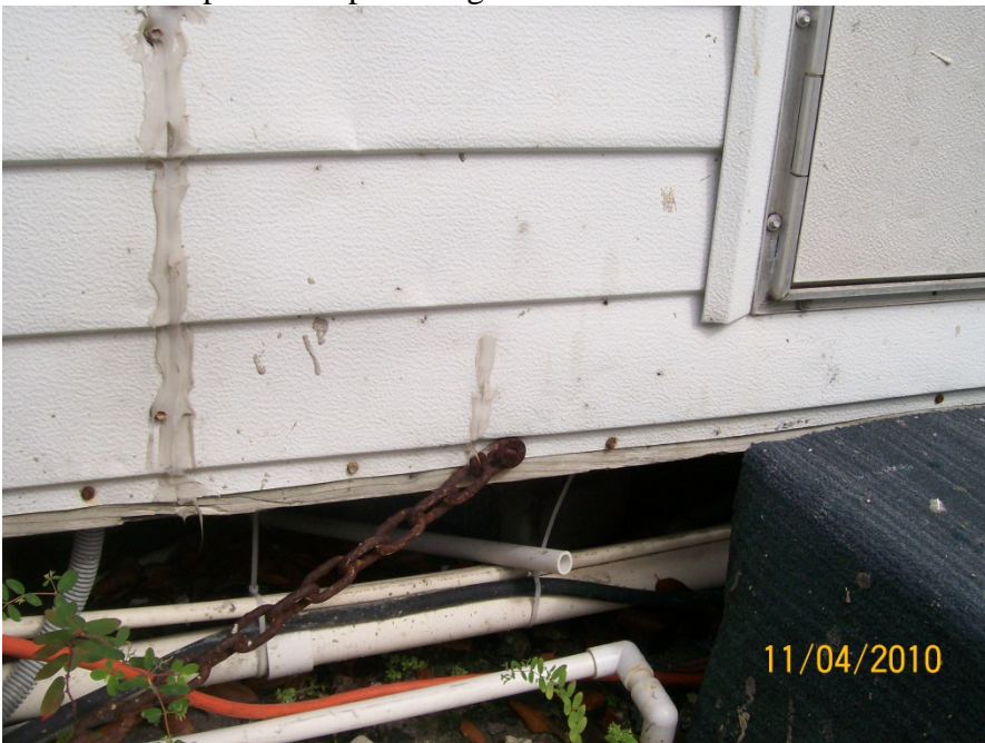
Photo #8 - Unpermitted plumbing work under shed #2 – left side of entrance door
