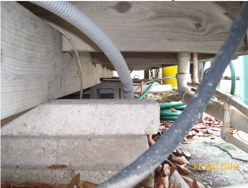
Photo #10 - Underside of 2 nd shed with cable and orange extension cord for electric leading from temp pole
