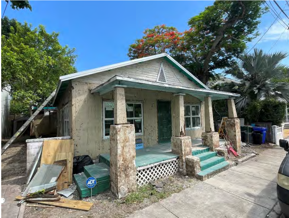
Photograph of the house without the stone veneer.
