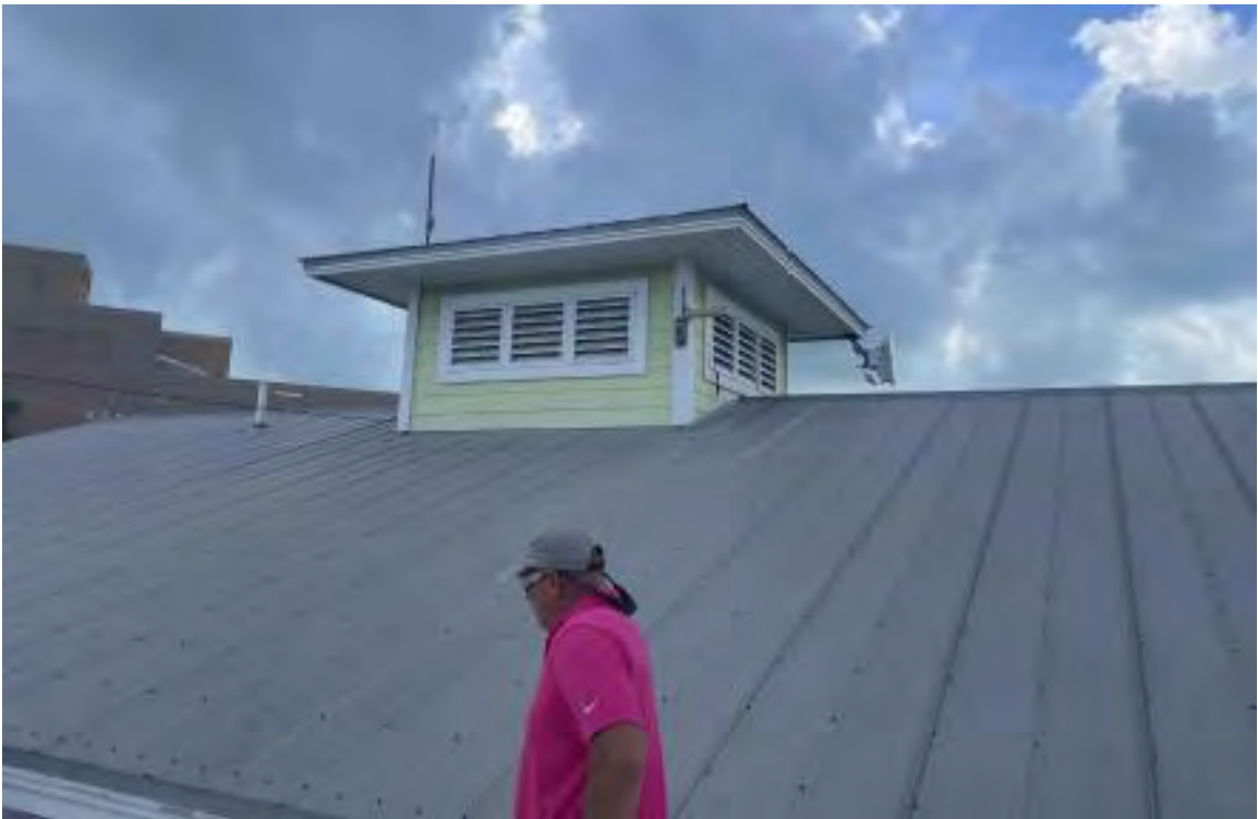
Photo of existing 5 V-crimp roofing system.
