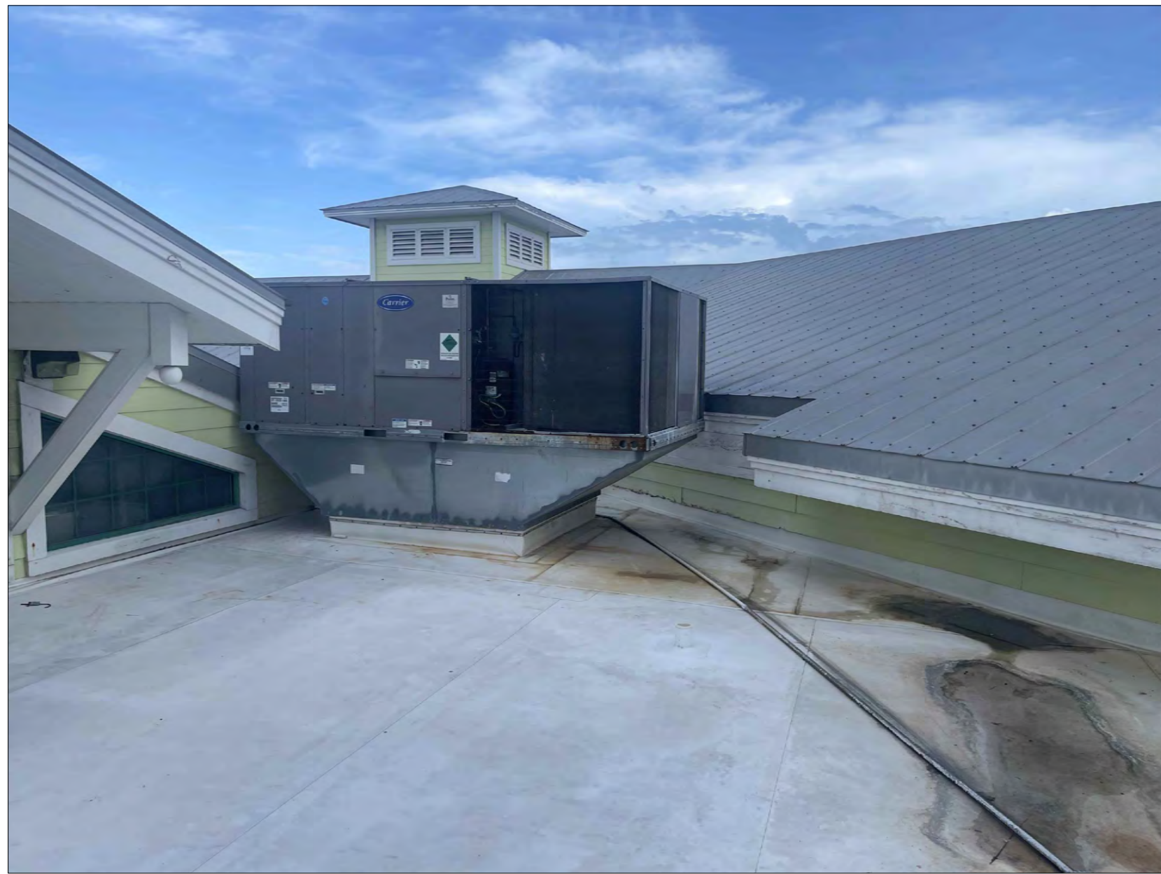
5 ROOF PHOTO EX2.2
