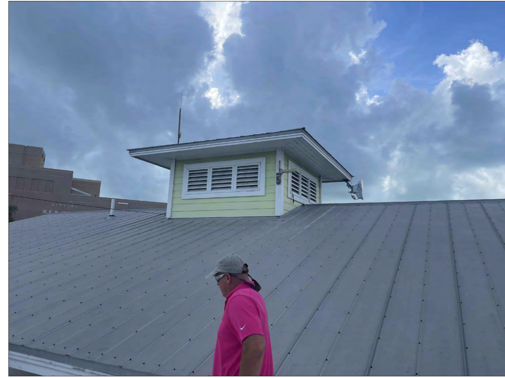
3 ROOF PHOTO EX2.2
