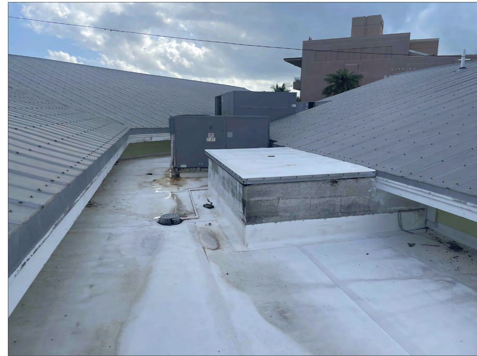
6 ROOF PHOTO EX2.2
