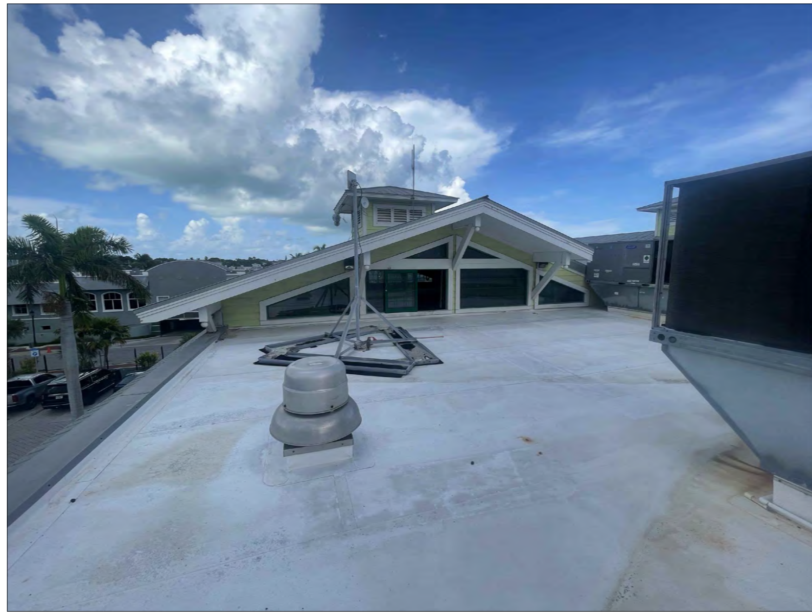
4 ROOF PHOTO EX2.2
