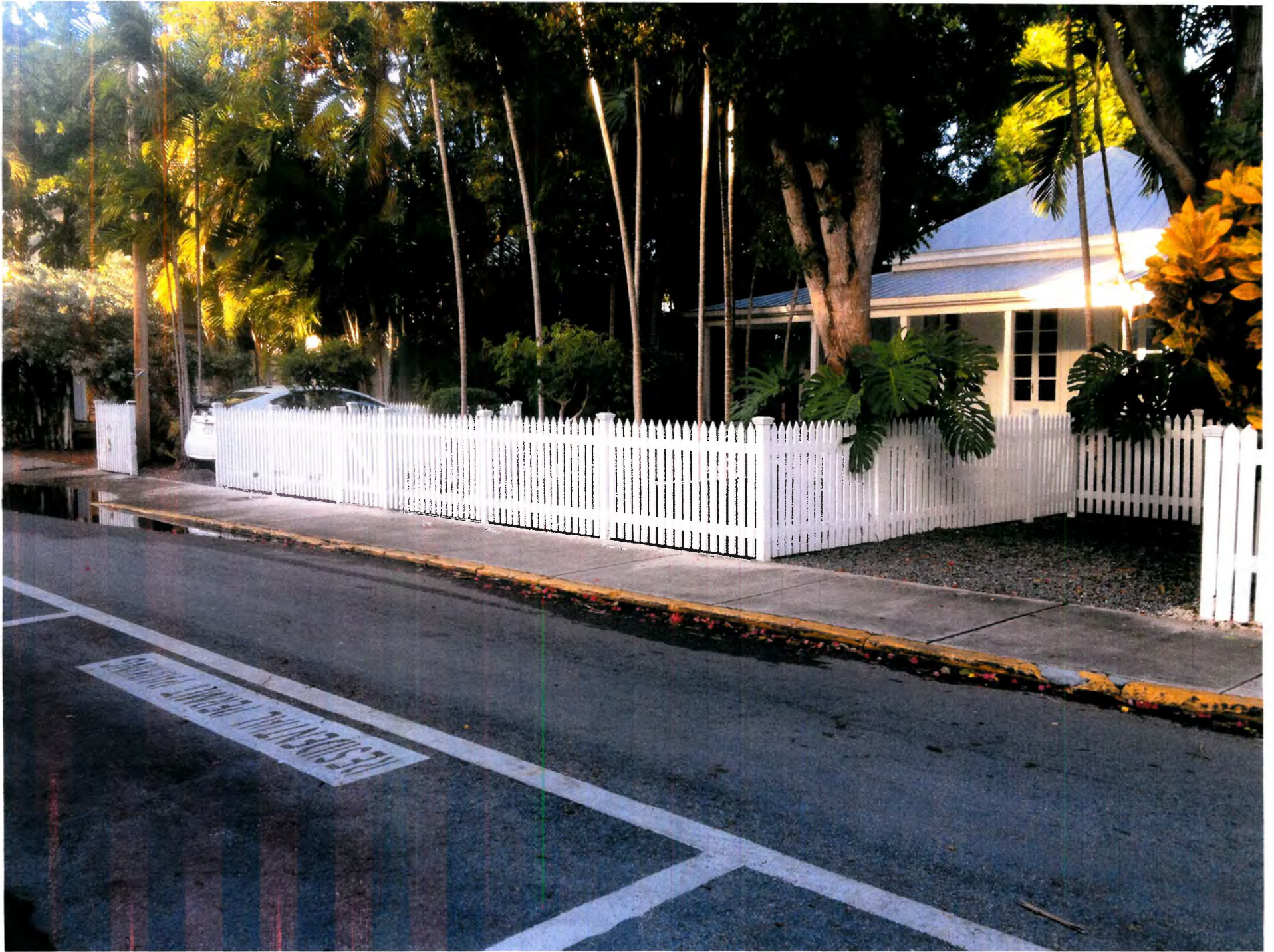
711 ASHE STREET VIEW FROM SOUTHWEST
