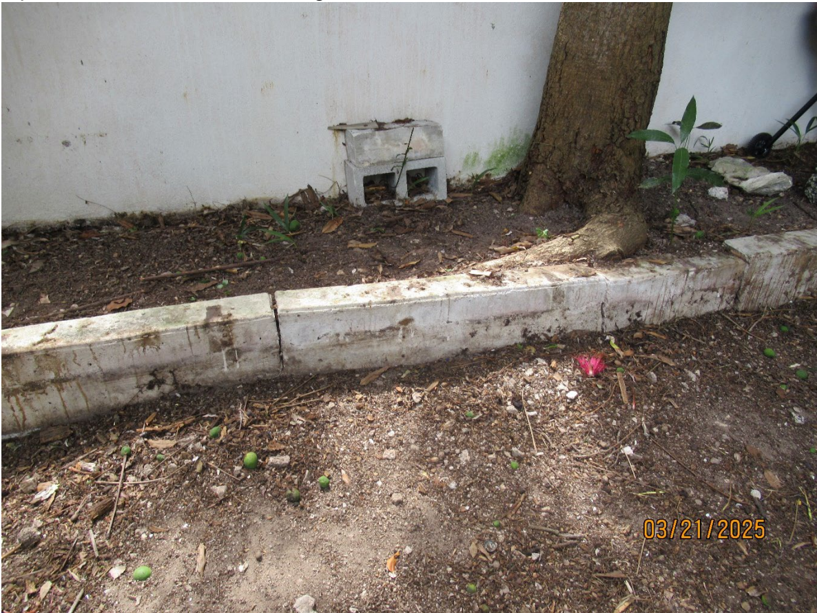
2 photos of the concrete cracking on the raised bed
