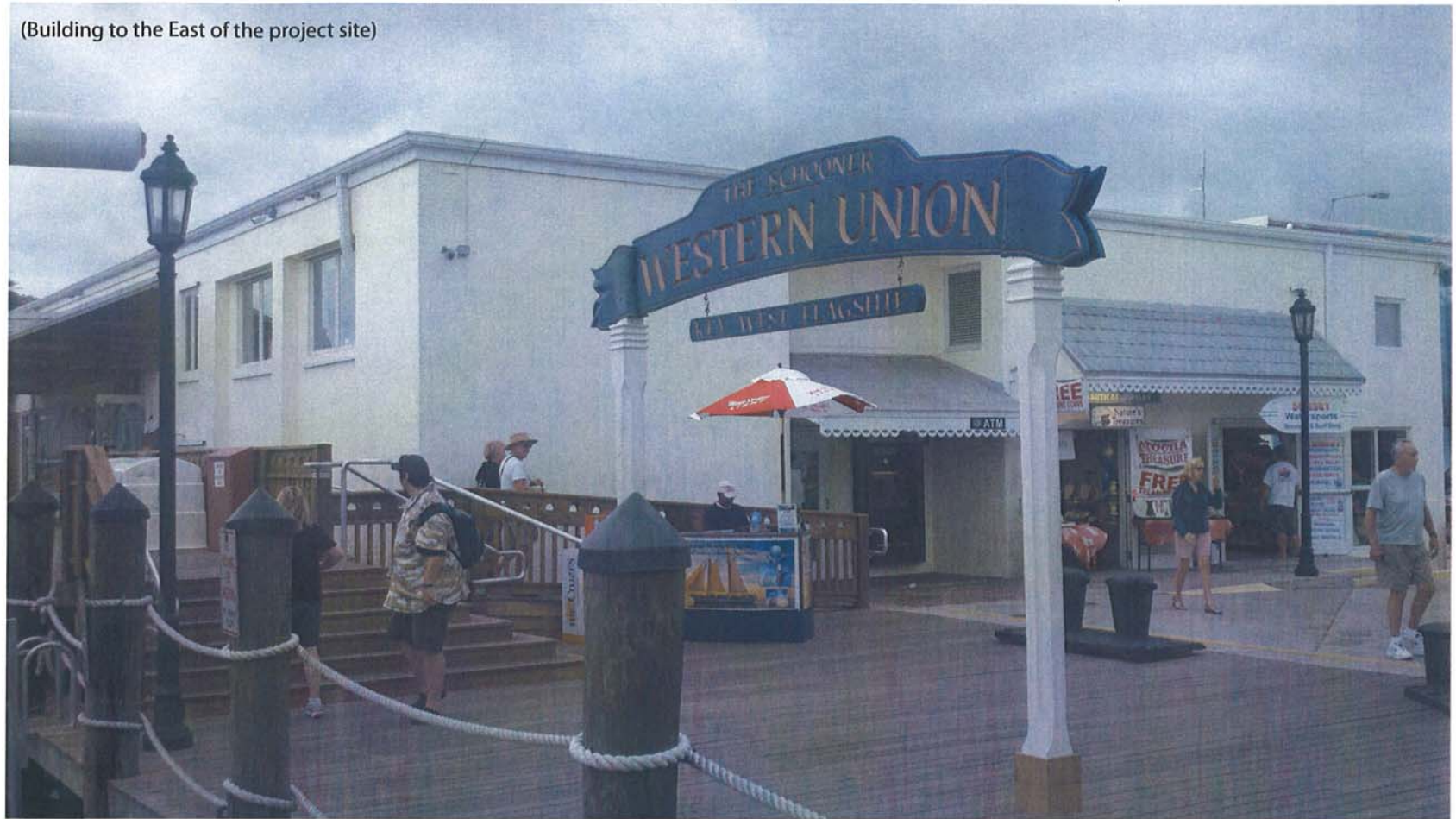
(Building to the West of the project site)
