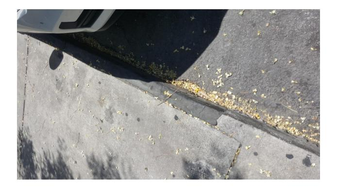
Figure 1-8. View of a Section of Historic Slate Curb on Northwest Side of Southard Street, Key West (AECOM June 2019)
