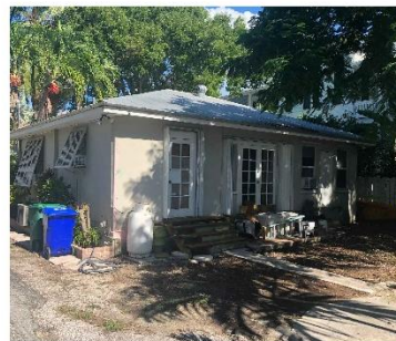
6 PHOTO OF 520 GRINNELL WEST EXTERIOR ELEVATION
