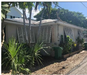
5 PHOTO OF 520 GRINNELL NORTH EXTERIOR ELEVATION
