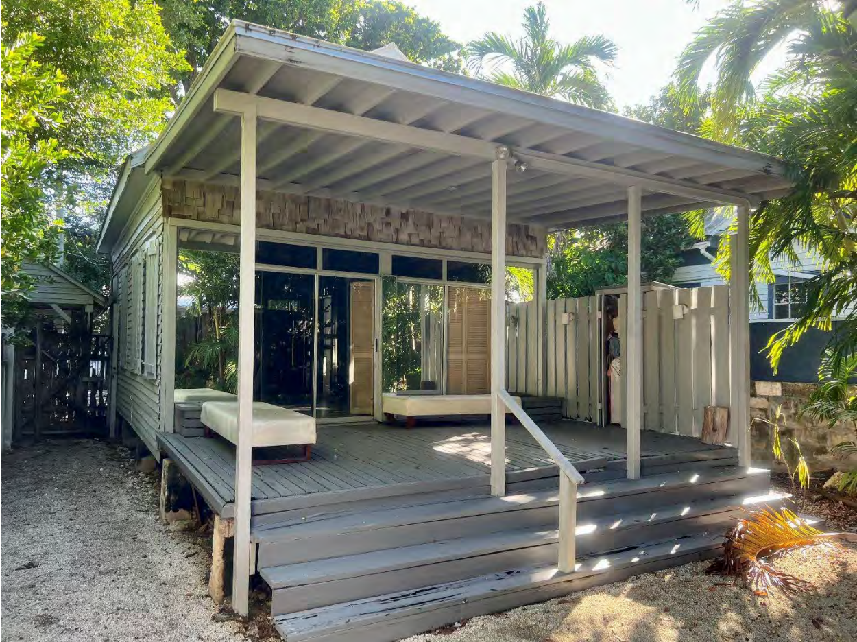
REAR AND NORTH SIDE
