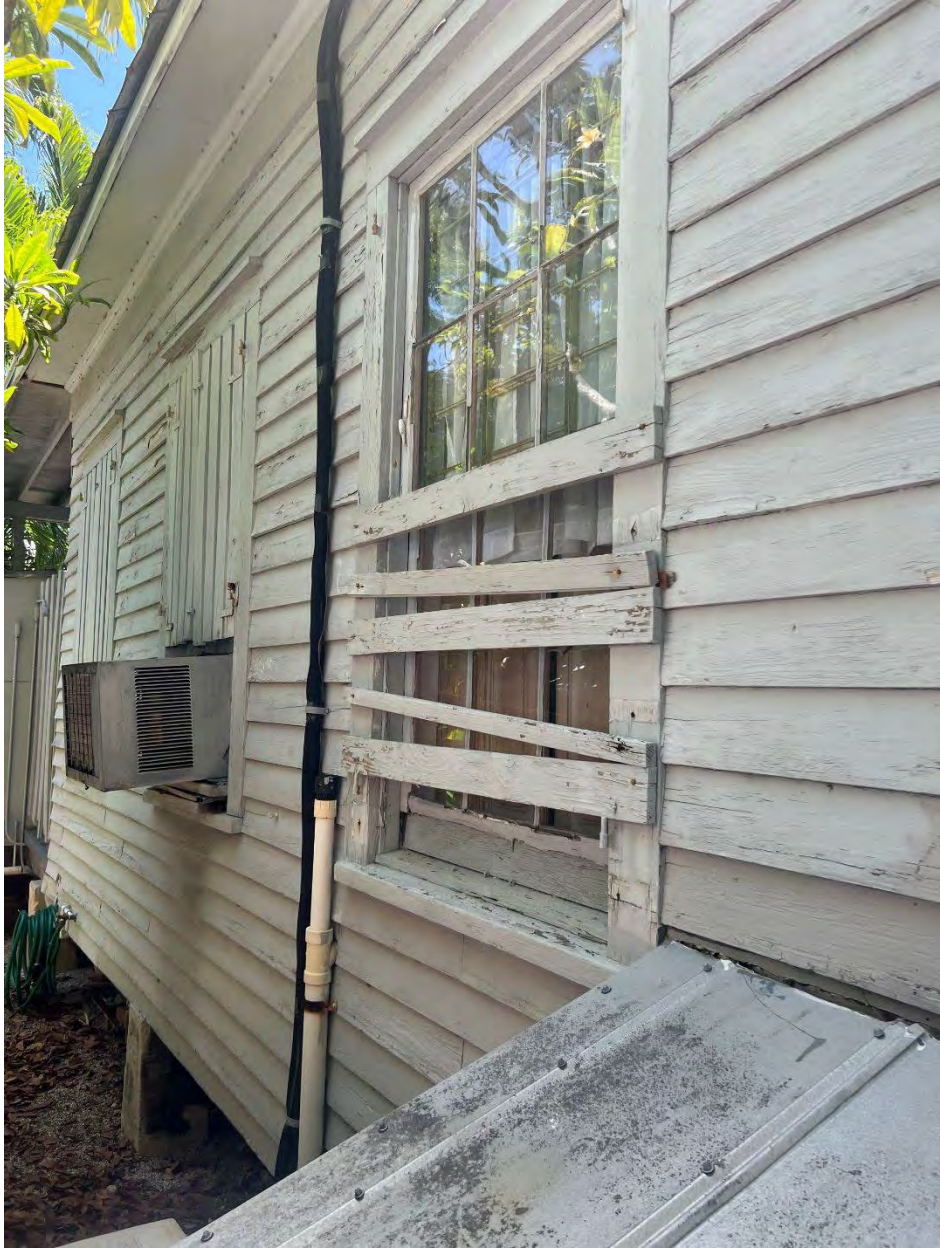
SOUTH SIDE OF HISTORIC STRUCTURE
