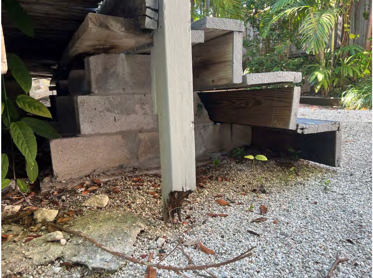
NON-HISTORIC REAR PORCH AND STEPS FOUNDATIONS
