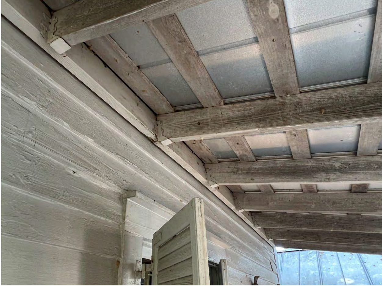
FRONT PORCH ROOF (ALTERED)
