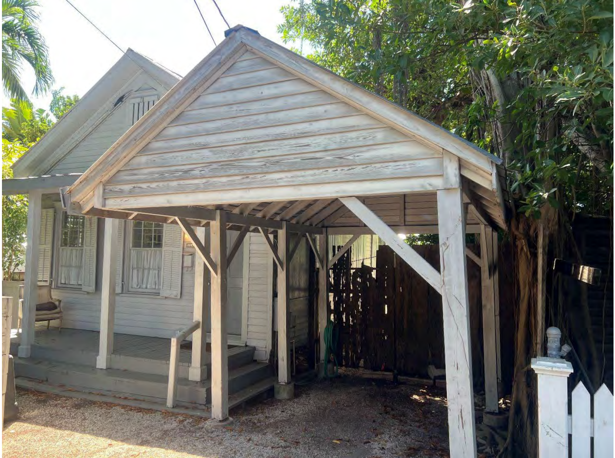
HISTORIC STRUCTURE AND CARPORT
