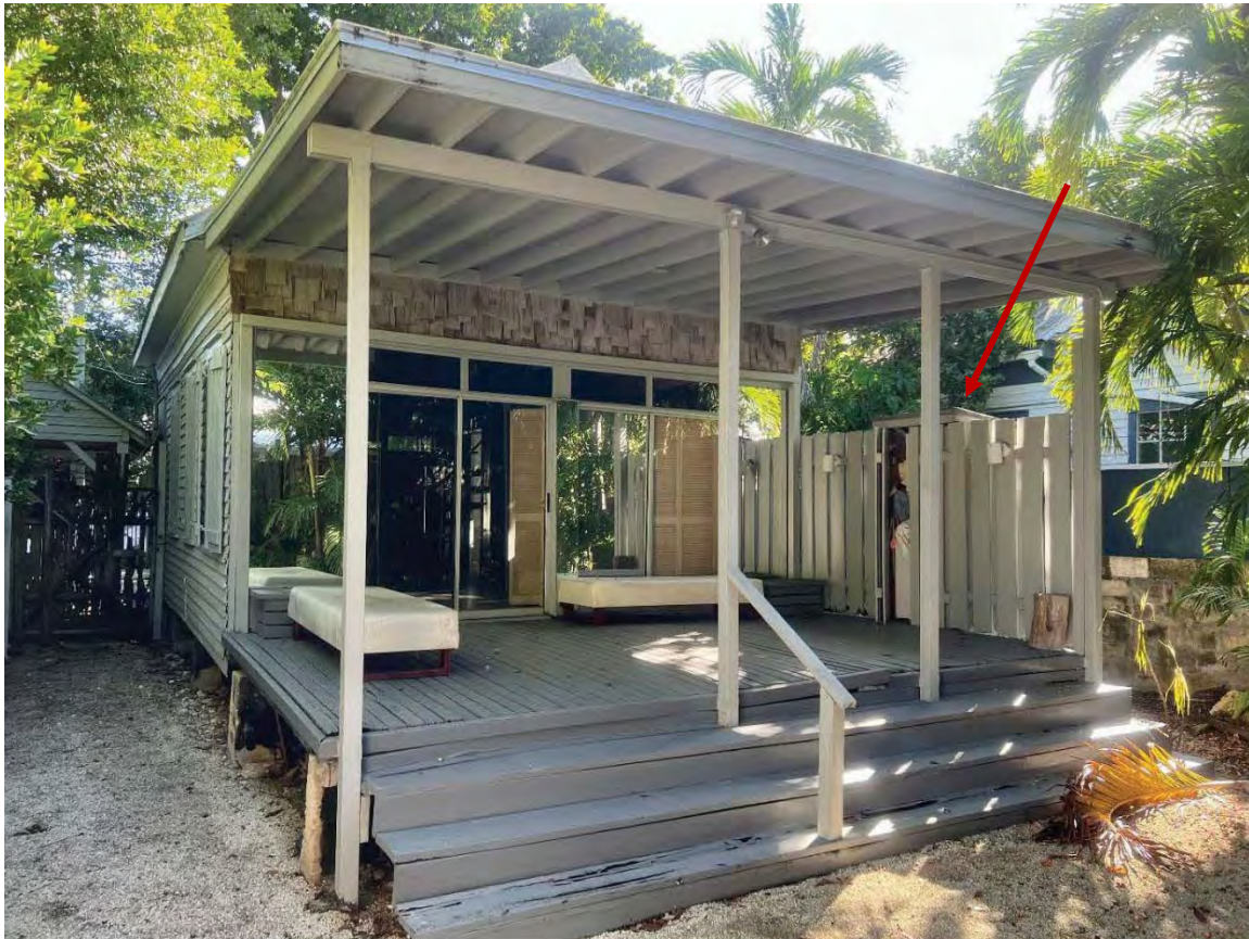
Rear View of The House. Arrow is pointing to the shed structure that is reflected as a bump-out in the existing street view elevation.
