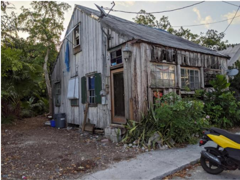
Front/side view of existing structure
