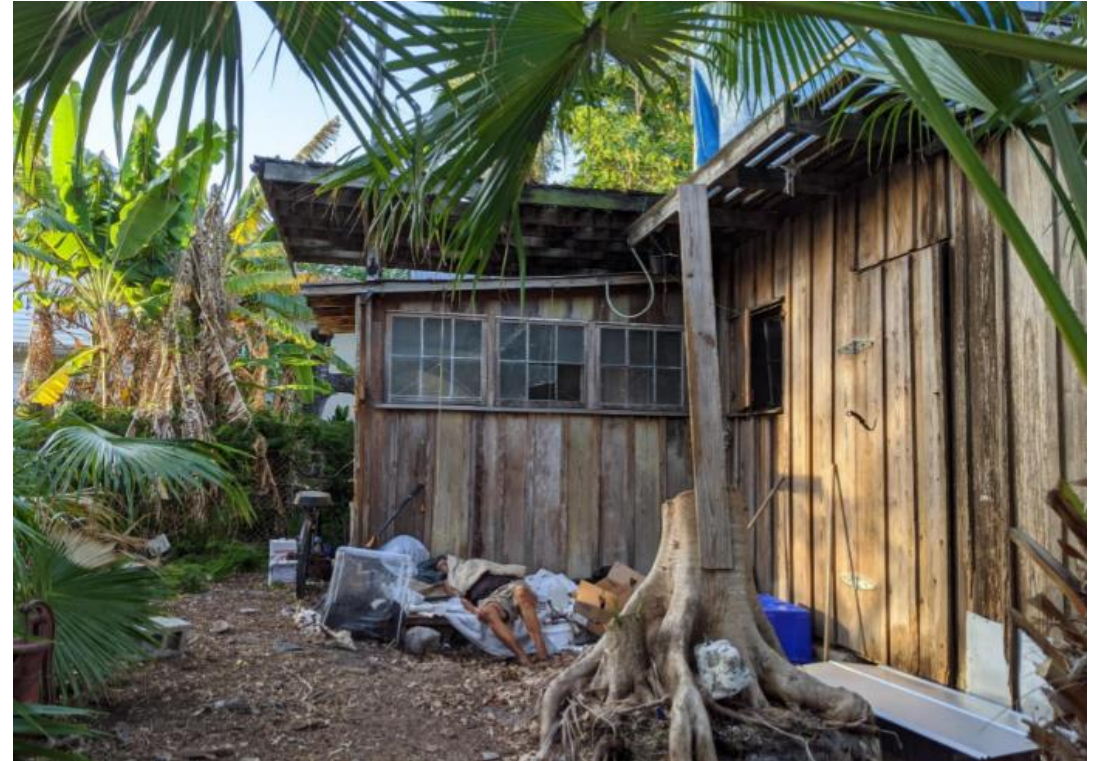
Rear view of existing structure
