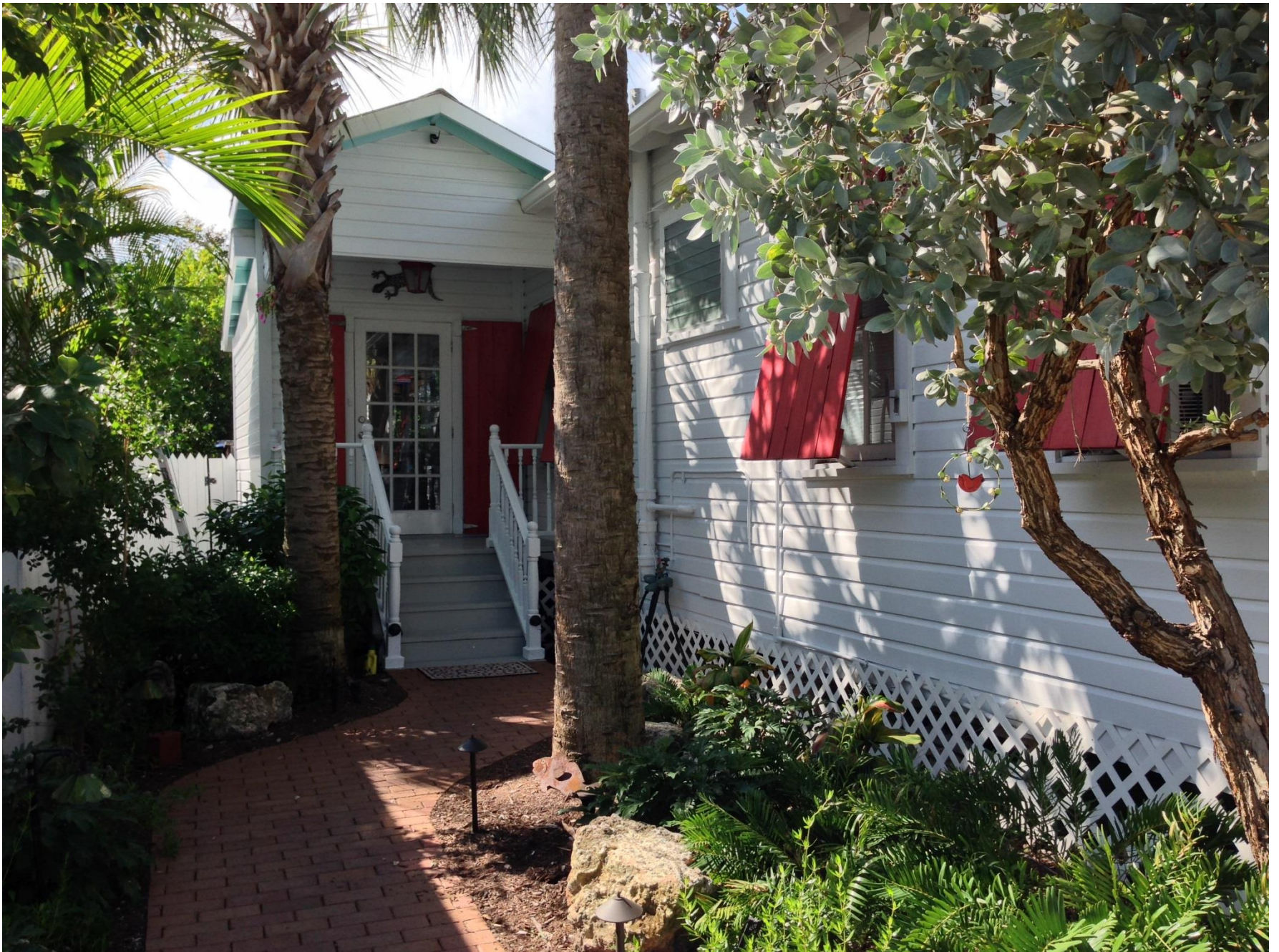
New main entranceway on left side of building.
