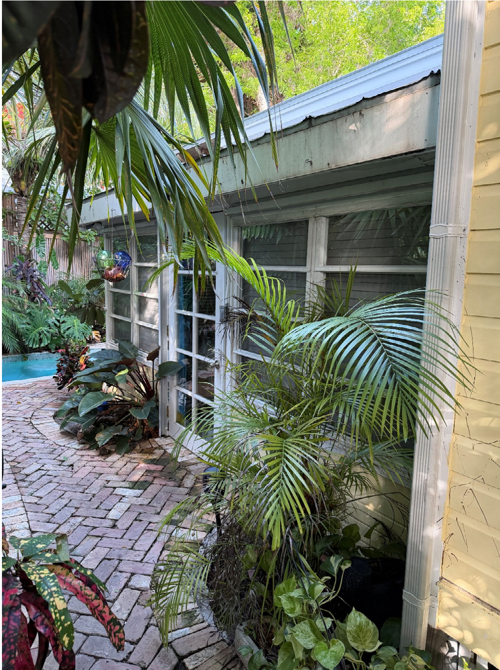
Figure 4 – Rear – North Side view of structure to be demolished
