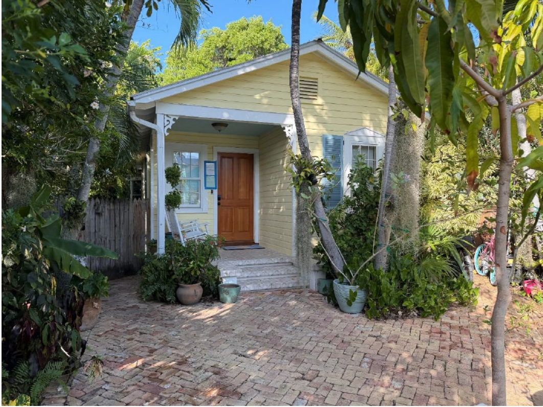
Photo of front of Property Under Review.
