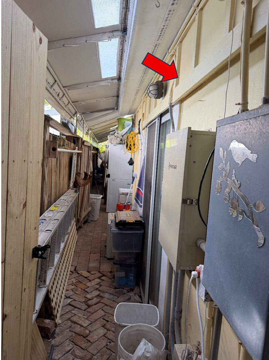
Figure 3 - South Side - viewed from Rear. CMU structure to remain indicated by red arrow
