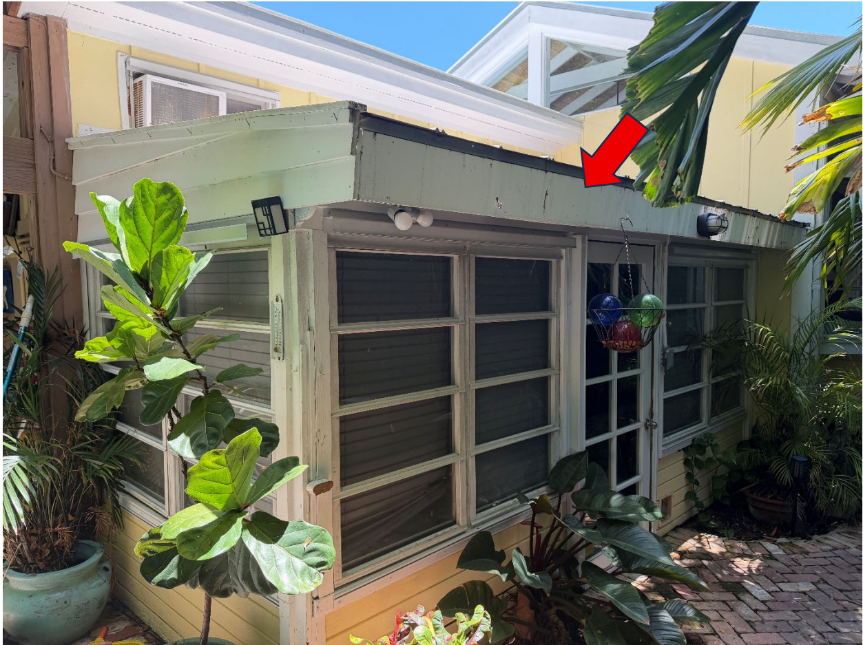
Figure 6 – Rear Corner view - Structure to be demolished indicated by red arrow.
