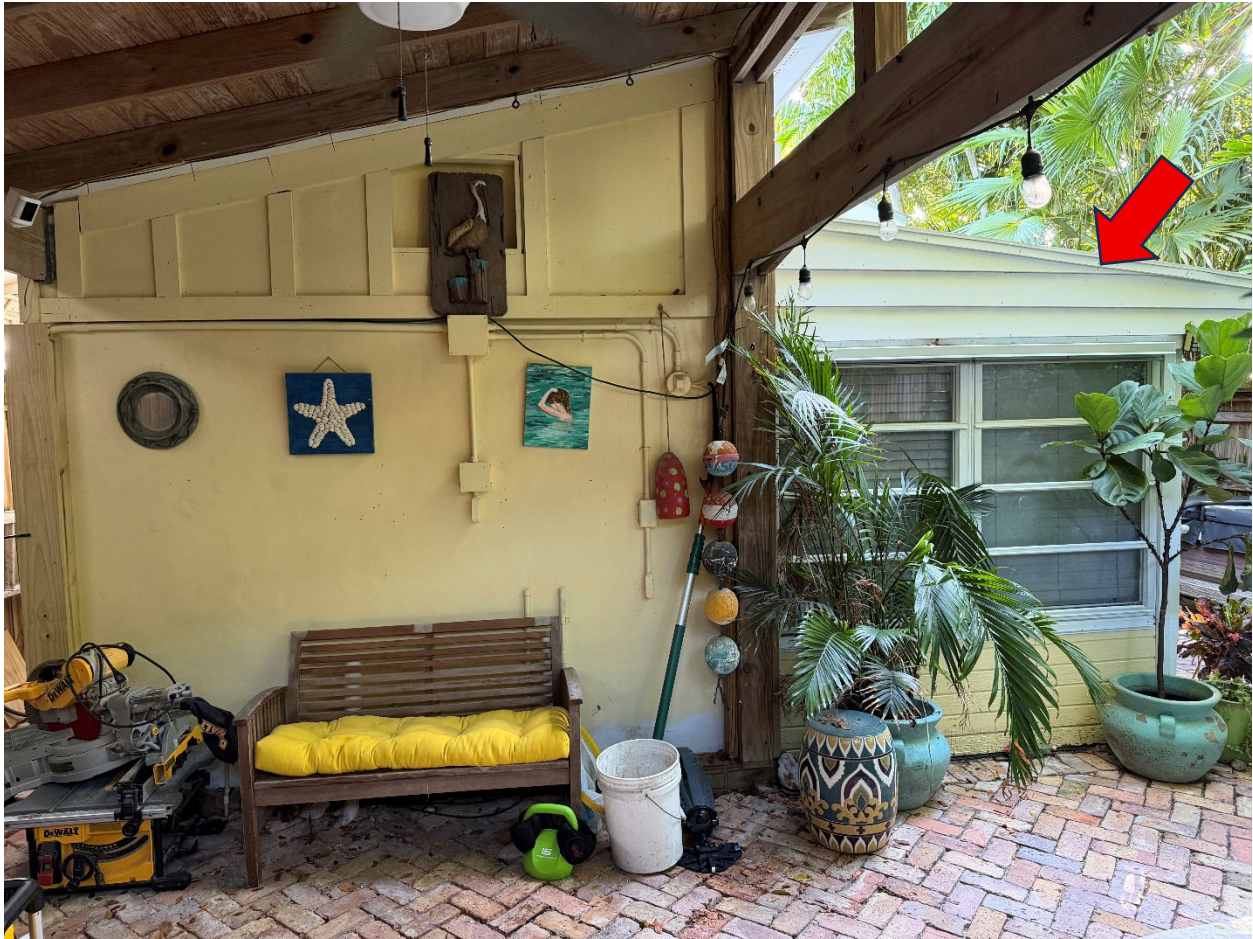
Figure 5 – Rear view, beneath open porch. Structure to be demolished indicated by red arrow.
