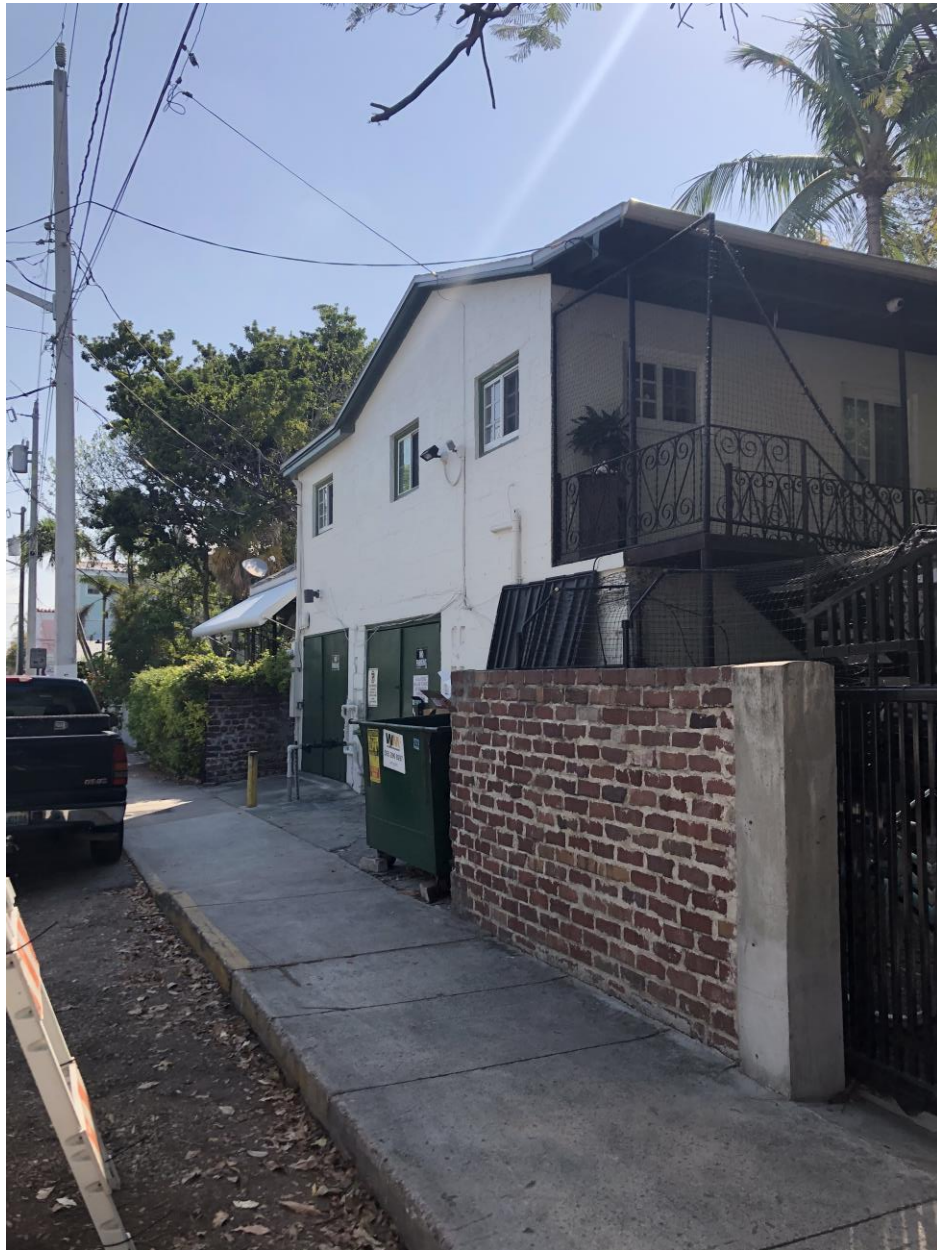
907 Whitehead Street- Photo dated April 16, 2021 – Exposed Trash Area
