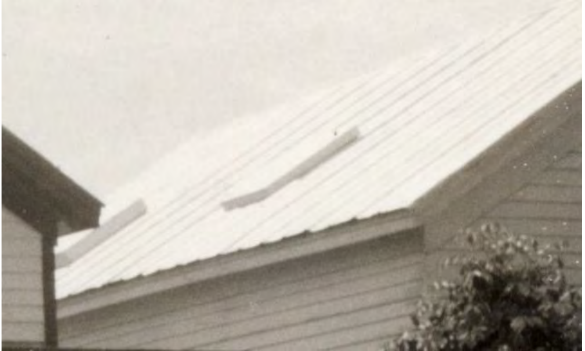
Detail of 1108 Fleming Street roof from circa 1965 photograph.
