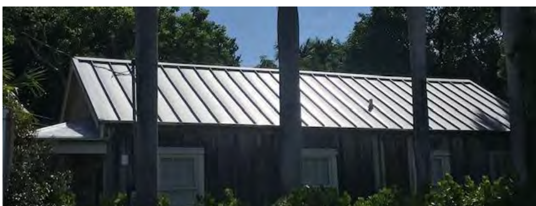
1400 Virginia Street after with standing seam.
