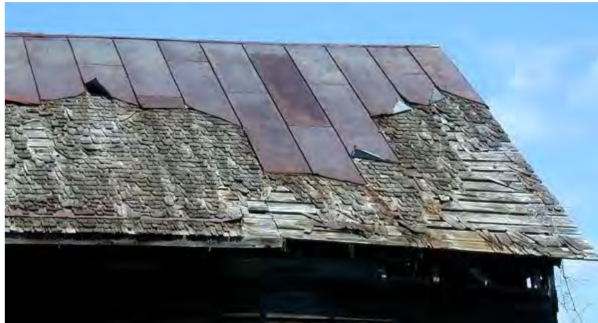
Example of a historic copper roof with standing seam.
