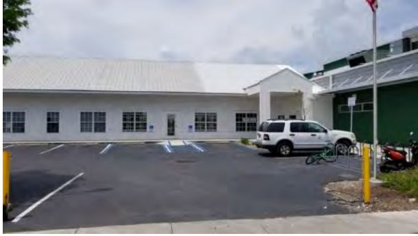
Subject Exterior – office building
