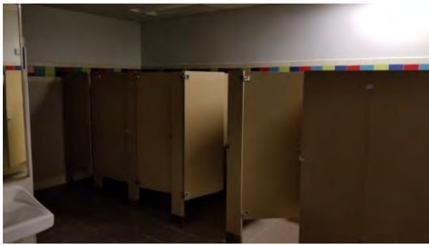
Interior of renovated gym – restroom
