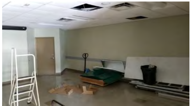
Interior of office space – single story building
