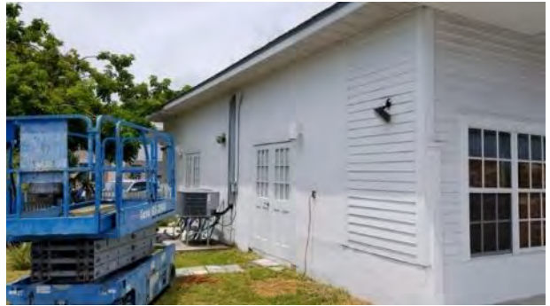
Subject Exterior – office building
