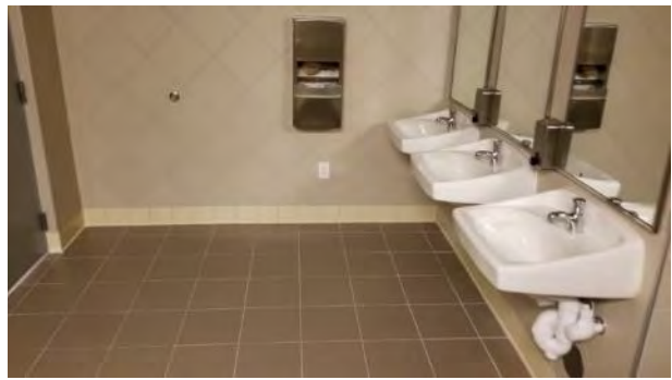
Interior of renovated gym - restroom
