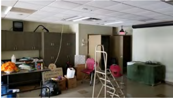
Interior of office space – single story building
