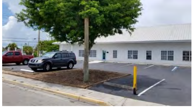
Subject Exterior – office building
