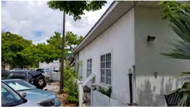
Subject Exterior – office building
