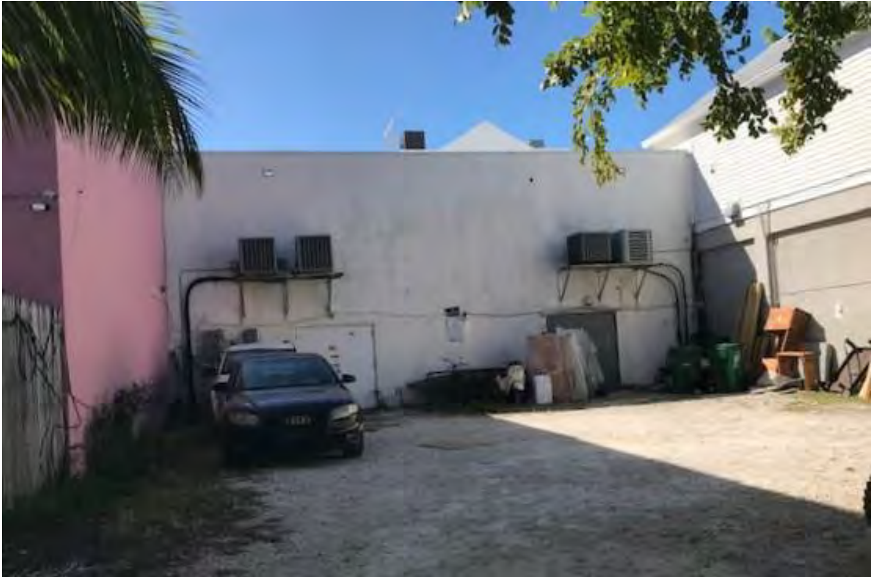
619 Duval Street REAR VIEW
