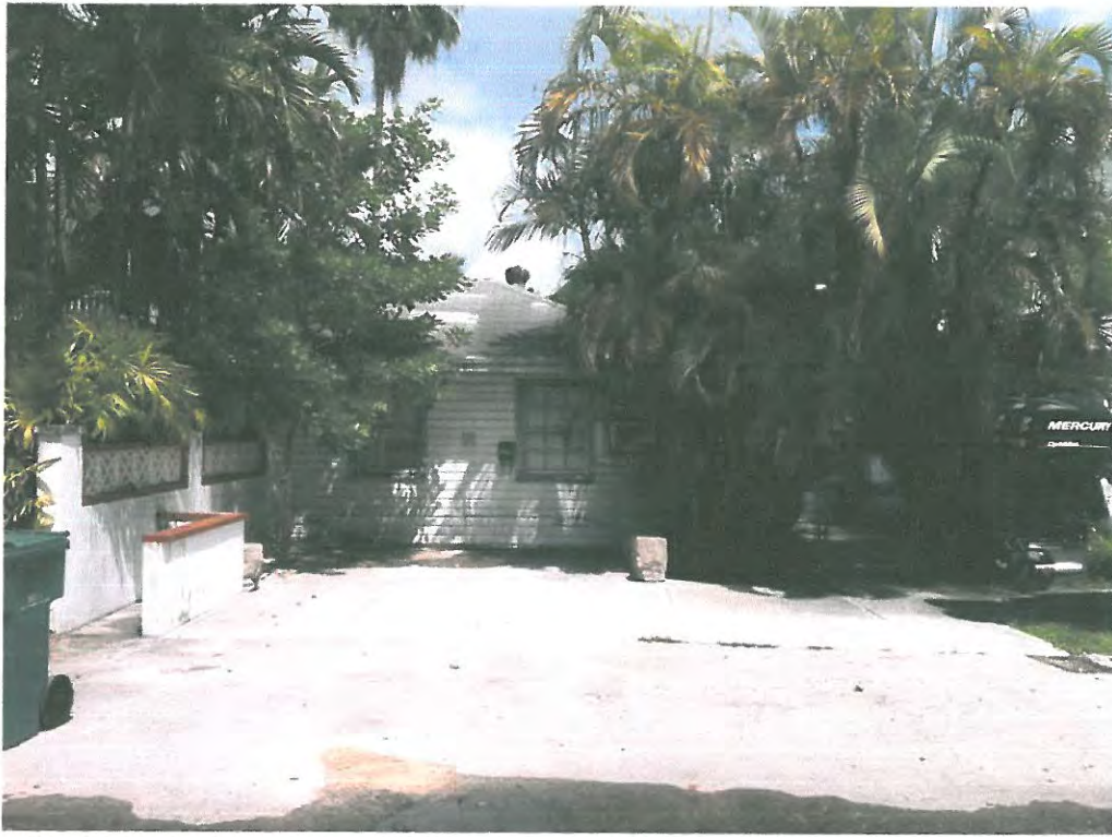
EXISTING HOUSE , 1133 VON PHISTER - FRONT VIEW
