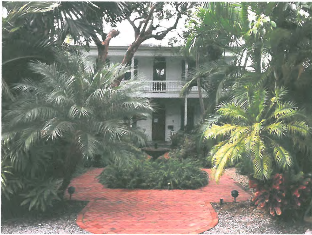
ADJACENT PROPERTY: 1131 VON PHISTER - FRONT VIEW
