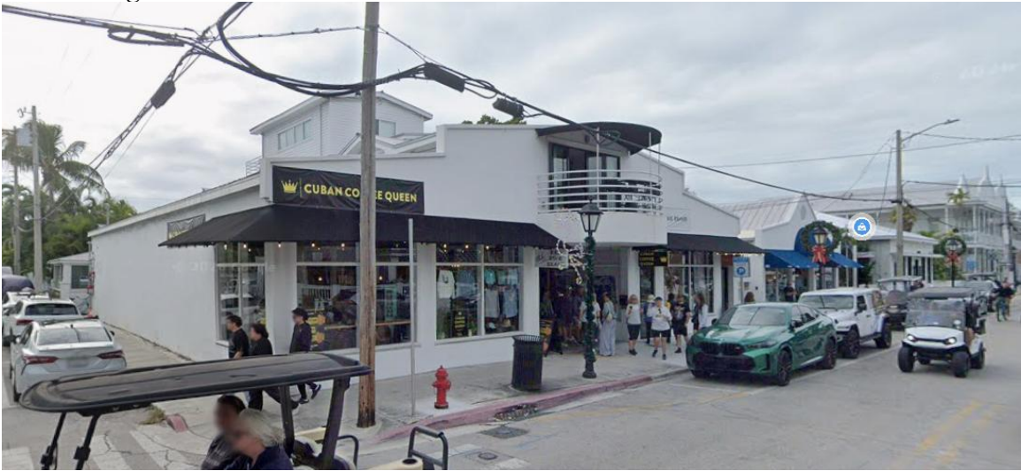
Cuban Coffee Queen - 1124 Duval Street: permitted in 2014 (no overhang) non-contributing structure.
