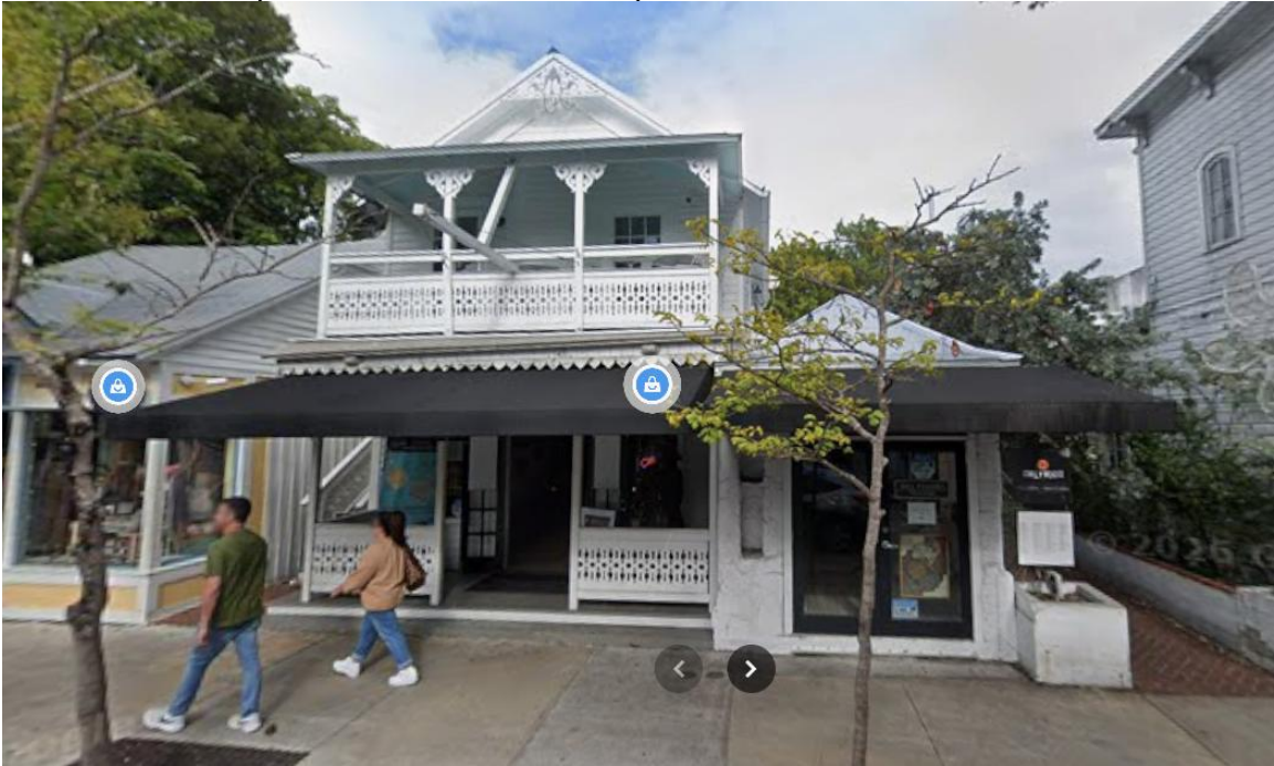
613 Duval Street: permitted in 1998, 2004 replacement, 2015 new over Mel Fisher's
