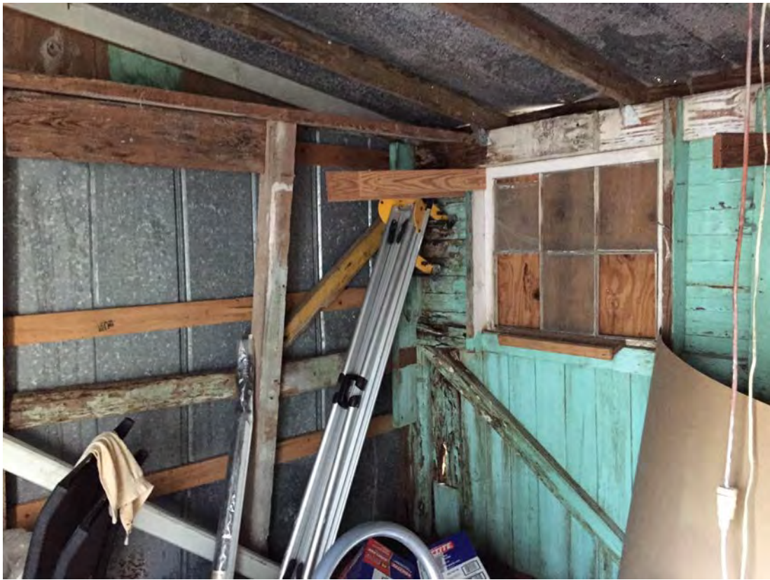
Interior of shed to be demoed
