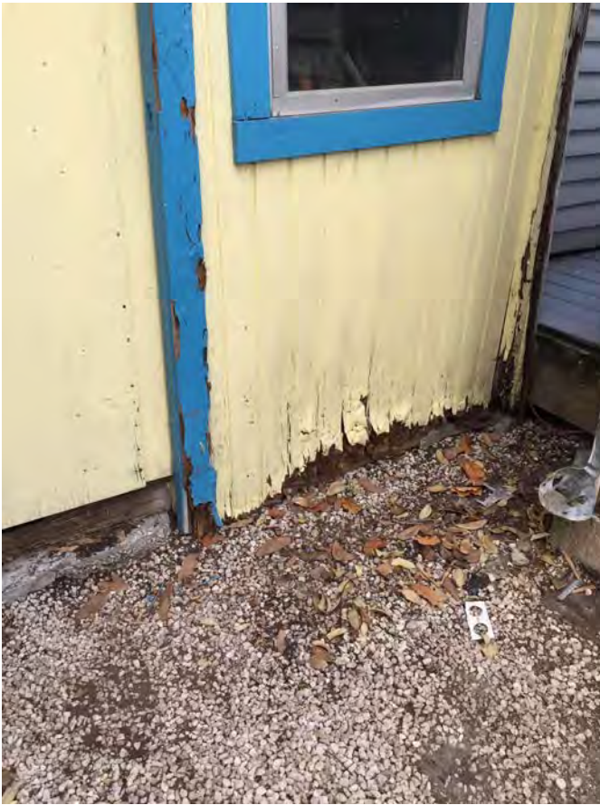
Shed to be demoed
