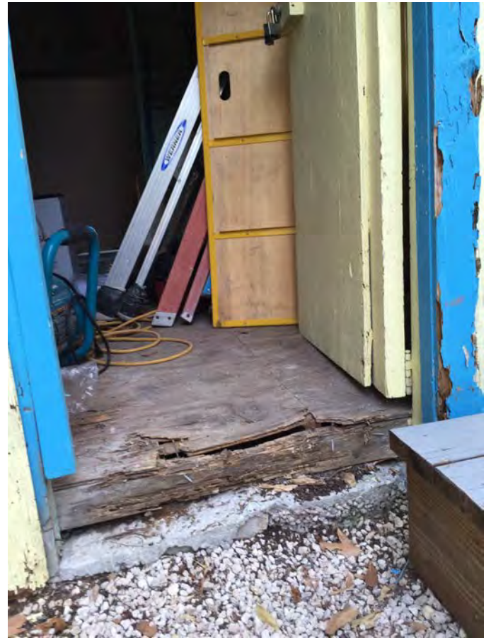
Shed to be demoed
