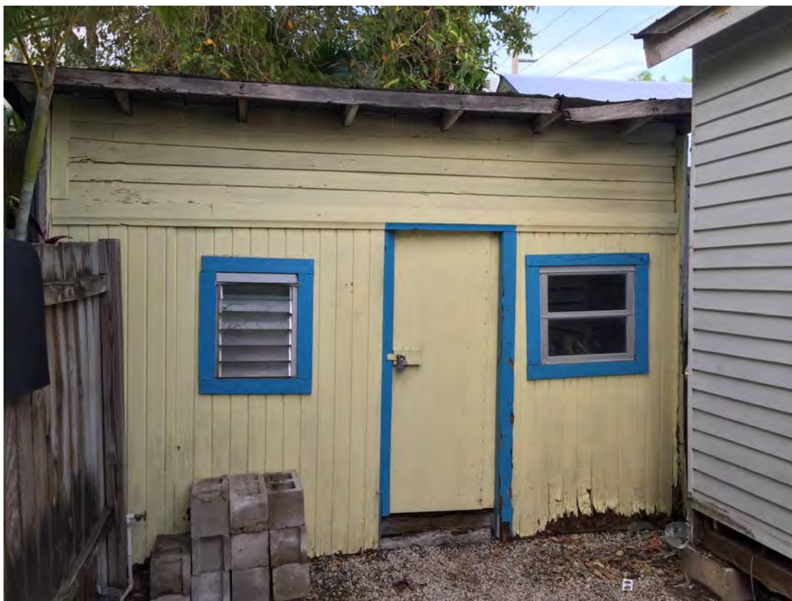
Shed to be demoed
