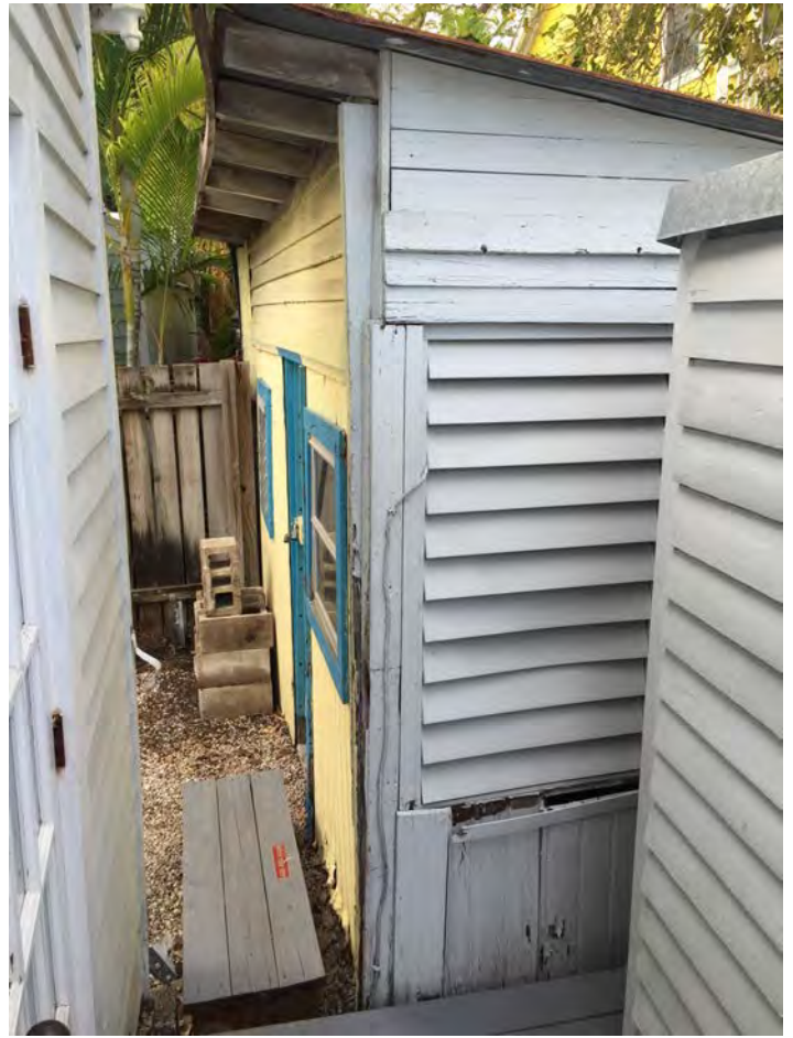
East Side Yard – shed to be demoed
