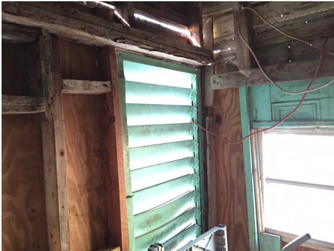
Interior of shed to be demoed
