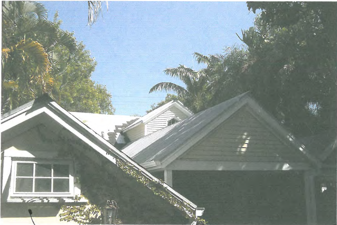
COTTAGE TO BE REMOVED
