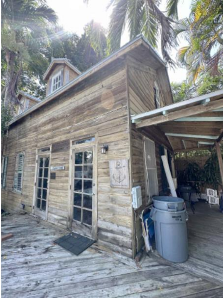
Photo of house under review before demolition.
