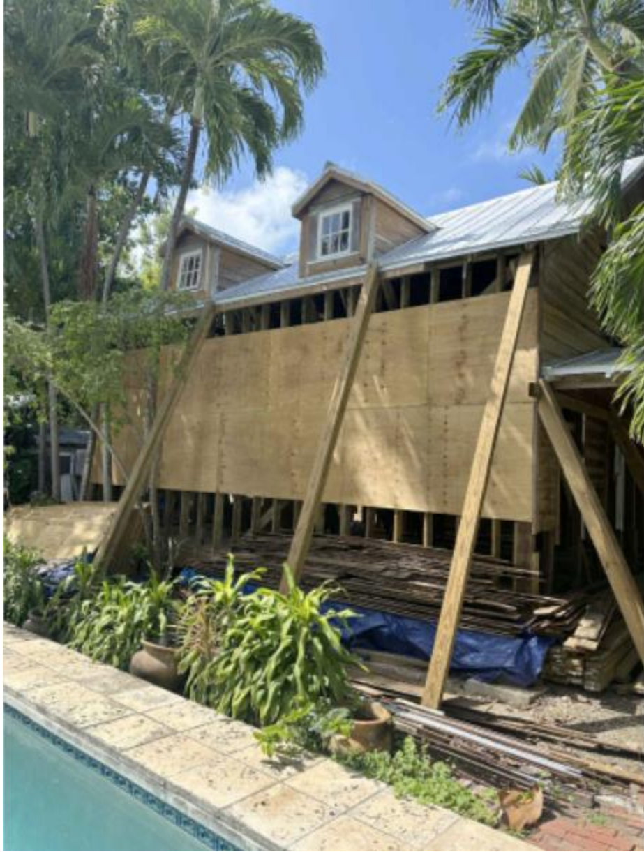
Photo of house under review after demolition.
