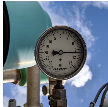
Figure 4-4. Blow Discharge Pressure Gauge
