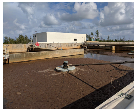
Figure 4-10. Post-anoxic Mixers
