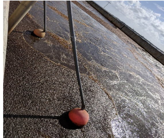
Figure 4-2. DO Probes in Bioreactors
