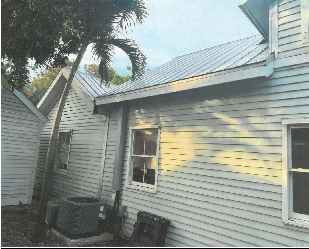
Area where the addition will be attached.
