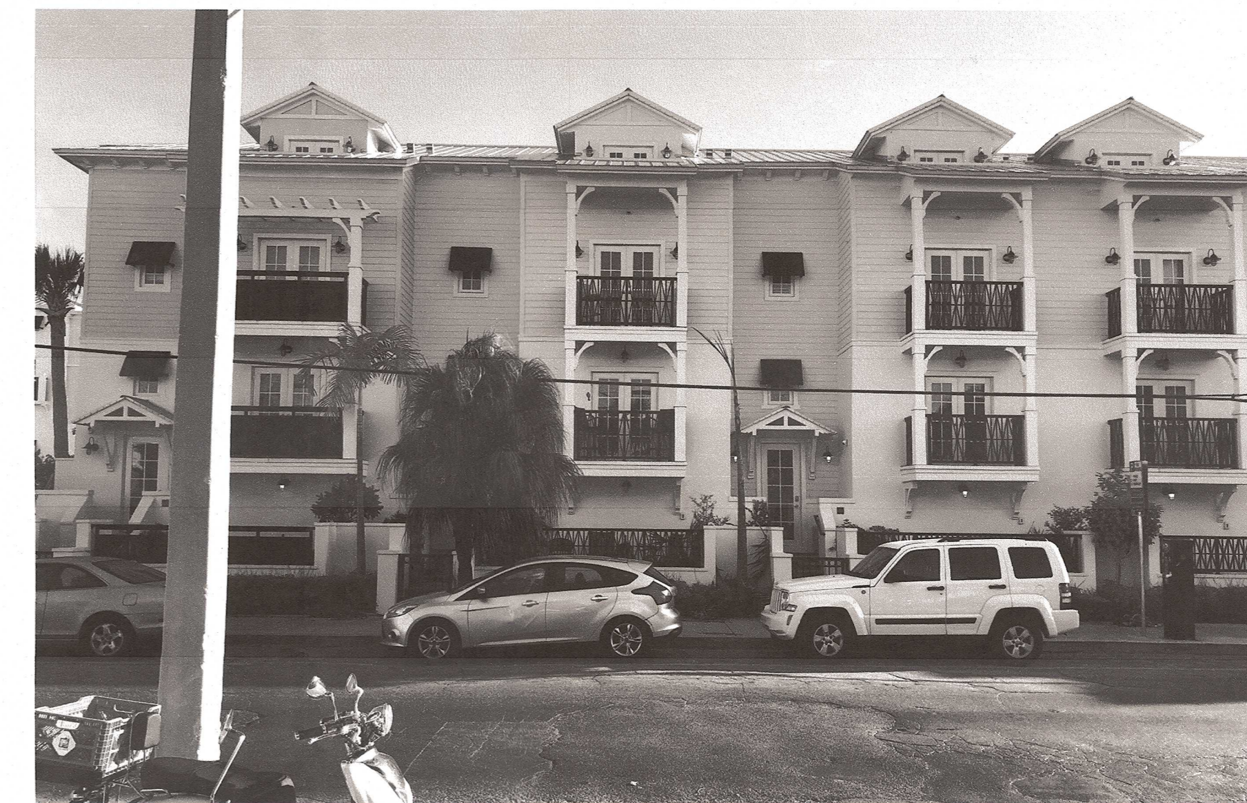
SAMPLE ELEVATION TAKEN AT 127-135 SIMONTON STREET (SAMPLE ONLY, INDICATIVE OF SIMILAR DETAILING, MATERIALS, AND COLORS)
