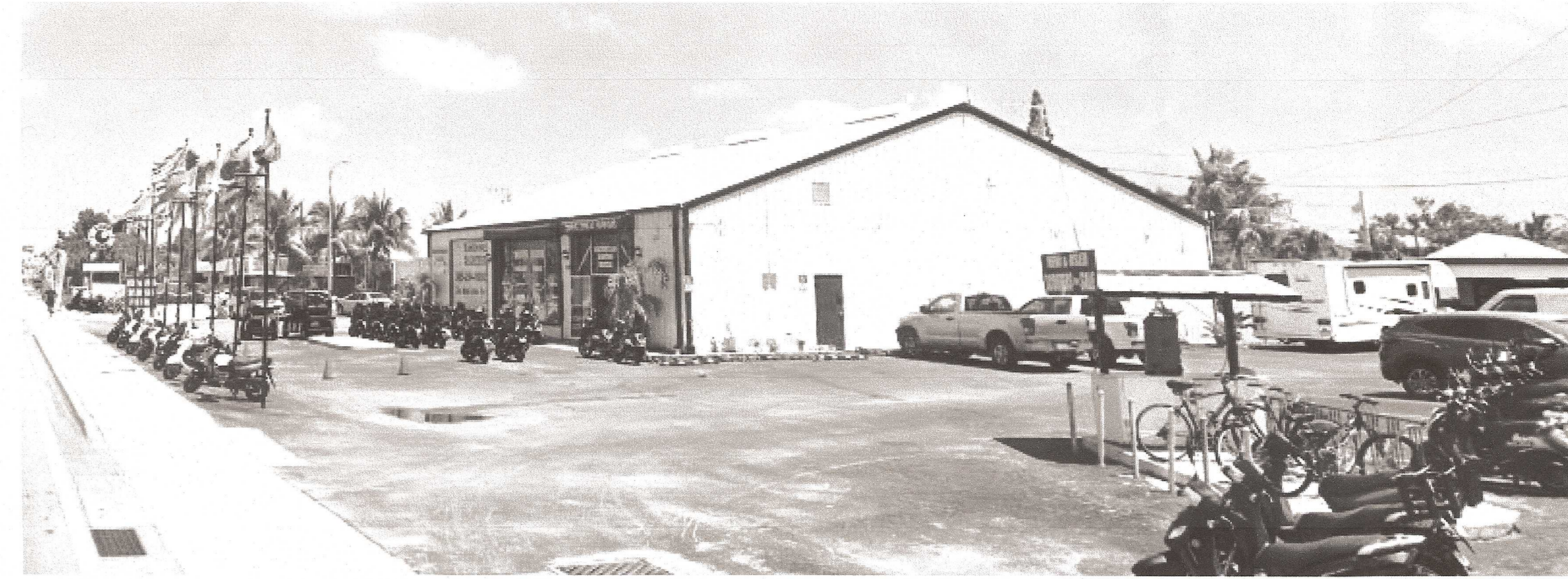
1910 N. ROOSEVELT BLVD. (TO BE DEMOLISHED)
