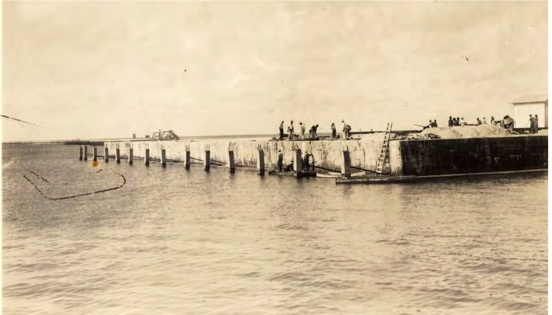
Pier B under construction circa 1930. Monroe County Library.
