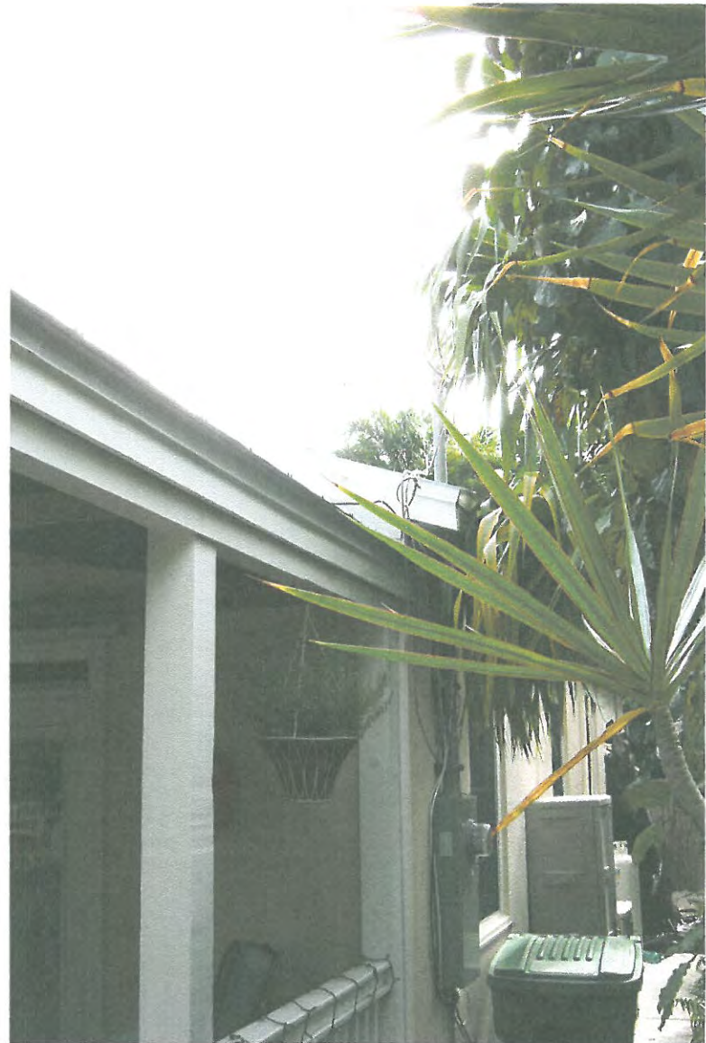
WEST SIDE LOOKING FRONT TO BACK
