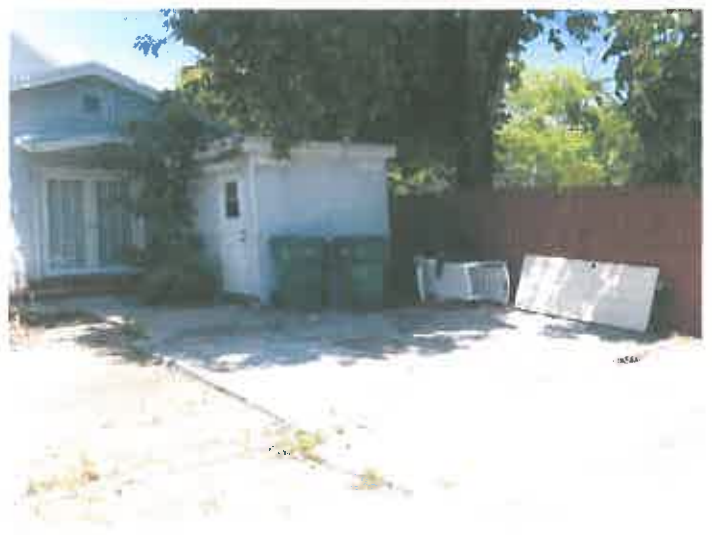
Shed and concrete to be removed
