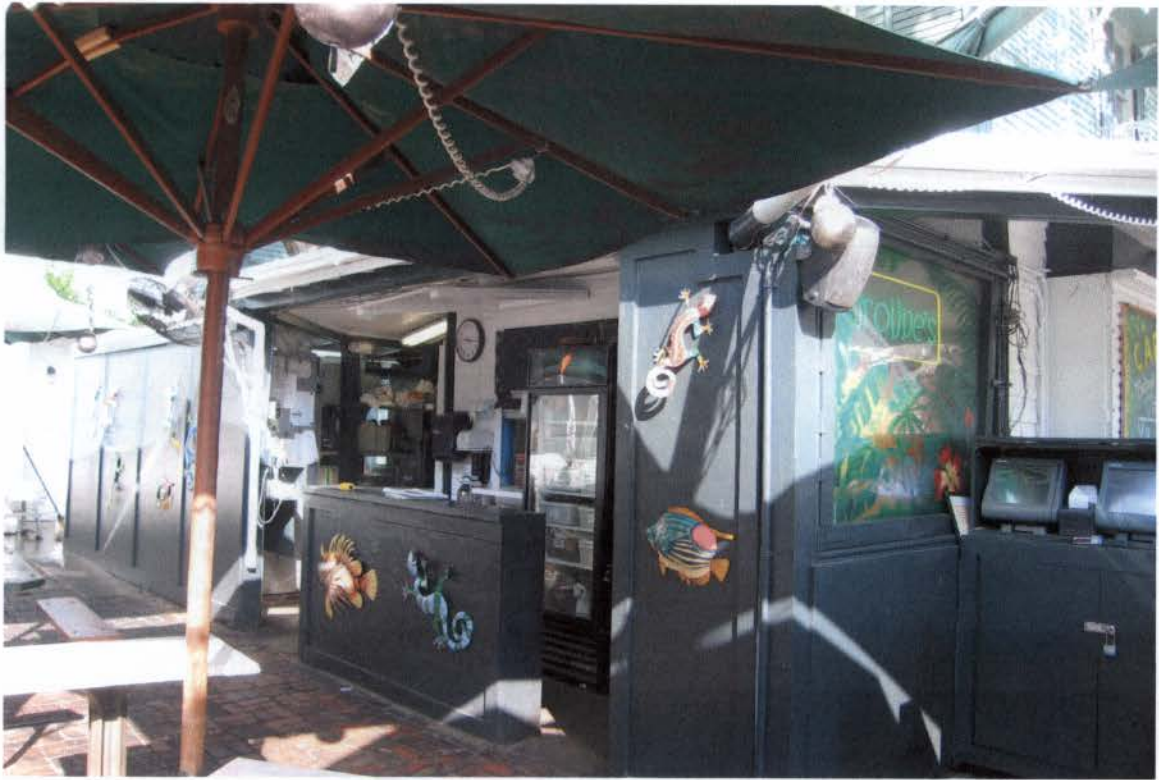
EXISTING KITCHEN BUILDING - SIDE VIEW
