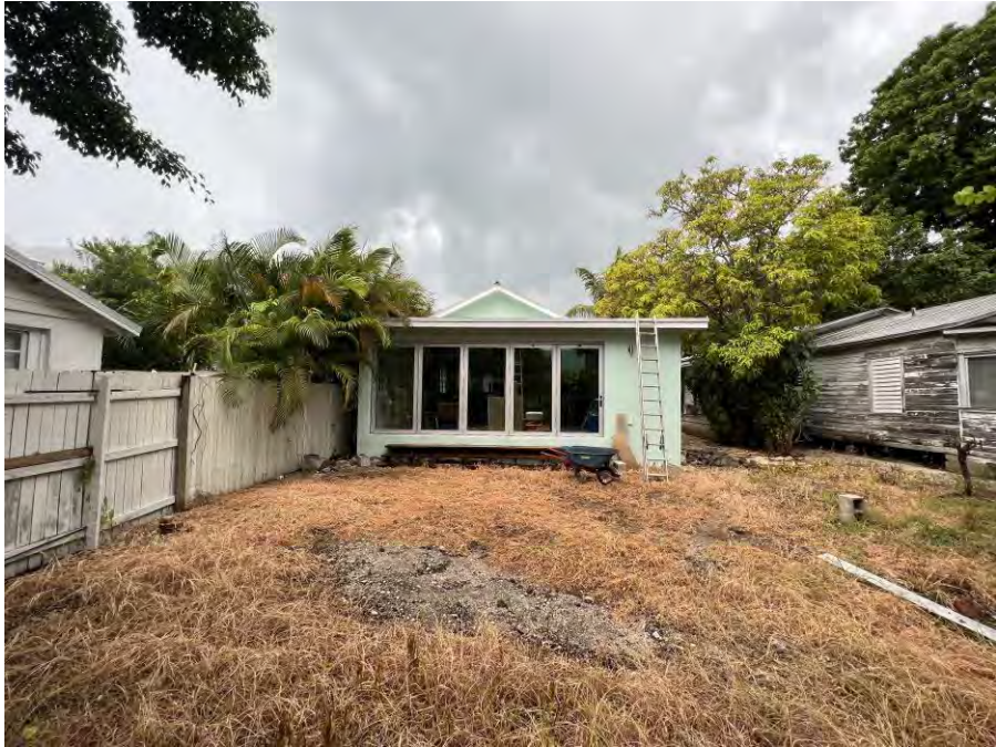
217 Eanes Lane – East Façade – Rear.
