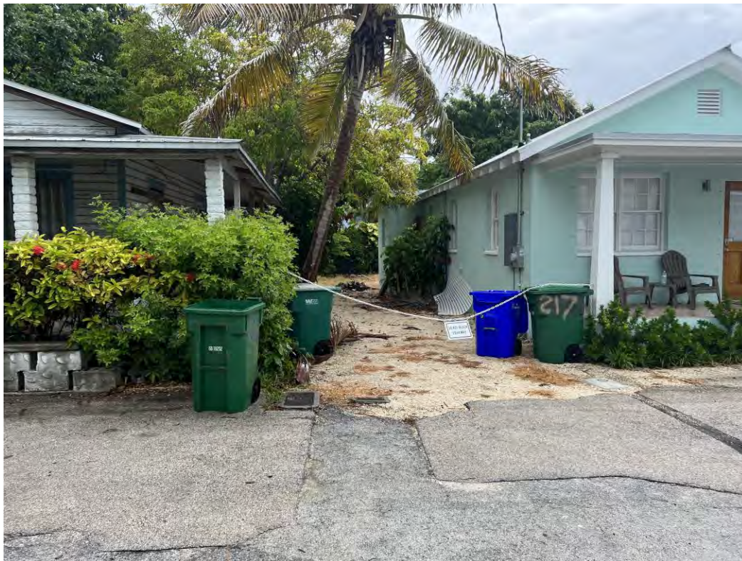
217 Eanes Lane – North Façade - Side.
